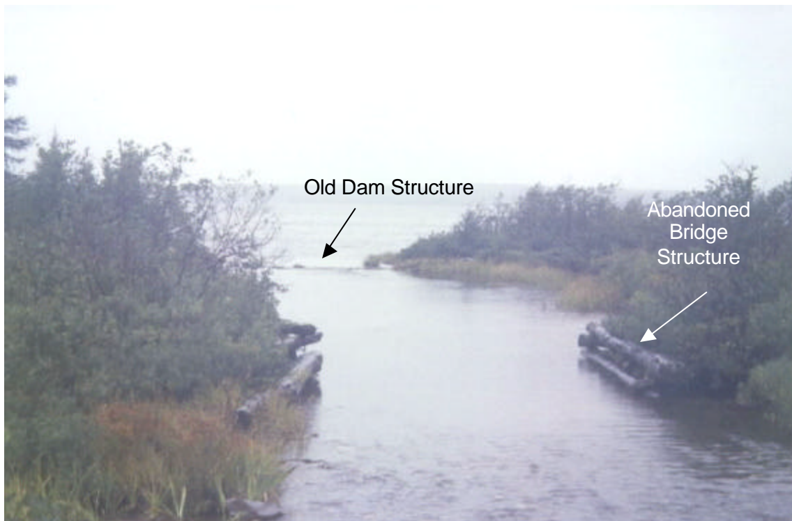
Figure 3.7. Tributary Three, the outflow of Andrew's Pond. The abandoned bridge/dam structure is visible.
