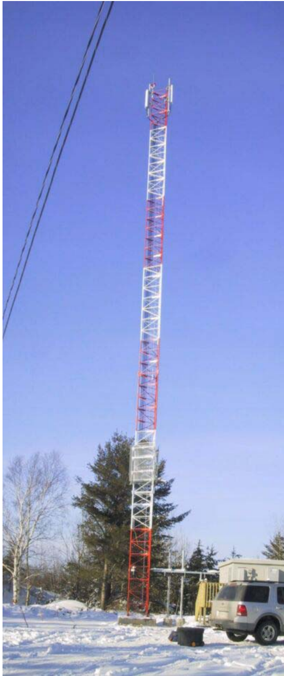
Typical Light Weight 30 m Self Supporting Communication Tower
