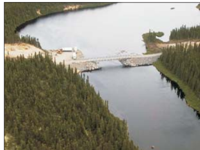
TEMPORARY BRIDGE ON THE GILBERT RIVER
