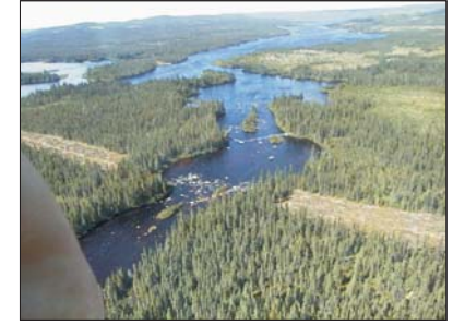
TEMPORARY BUFFER ZONE AT WATERCOURSE CROSSING
