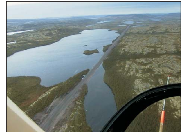
COMPLETED SECTION OF TRANS LABRADOR HIGHWAY - PHASE II
