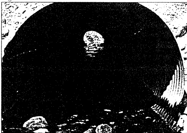
Figure 3. Countersunk Culvert
