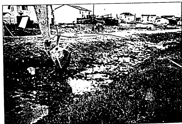
Instream excavation for stream crossing.
