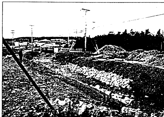
Stream crossing completed.
