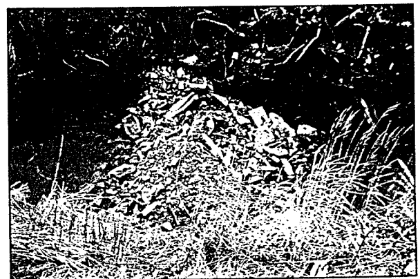
Ditch block (rock dam) used for low point protection.
