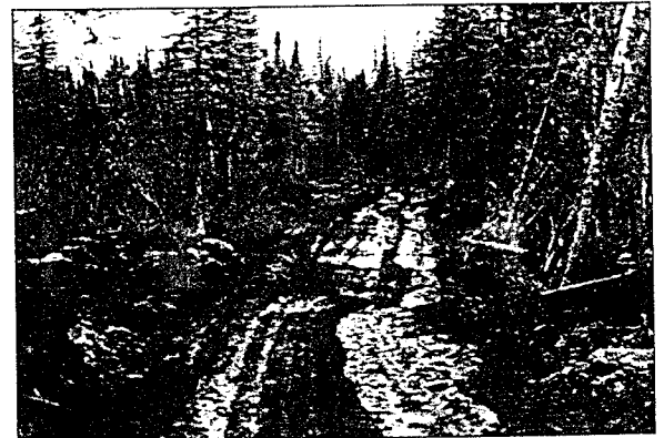
Poorly constructed access road.
