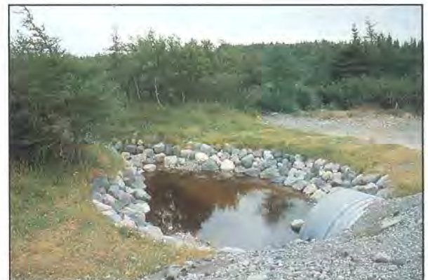
Rebuilt stream banks - rip rap, sod and natural vegetation.
