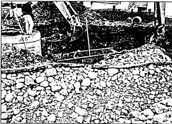
Stream bed restored.
