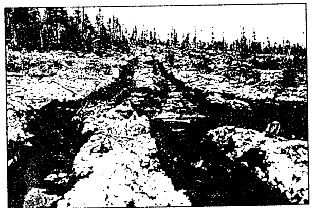
Mudlogs deflect water off the forwarder trail and unto the forest floor.
