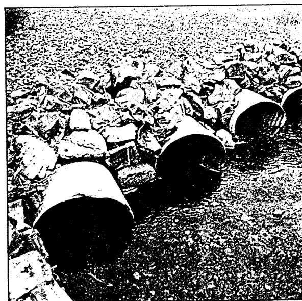
Stabilization of culvert outlets - rip rap.
