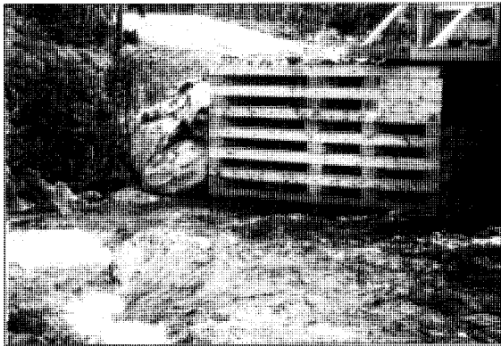
Timber crib construction: untreated/pressure treated wood.
