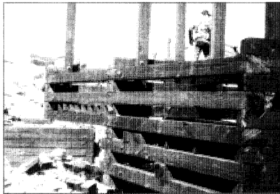
Timber crib construction for marine environment.
