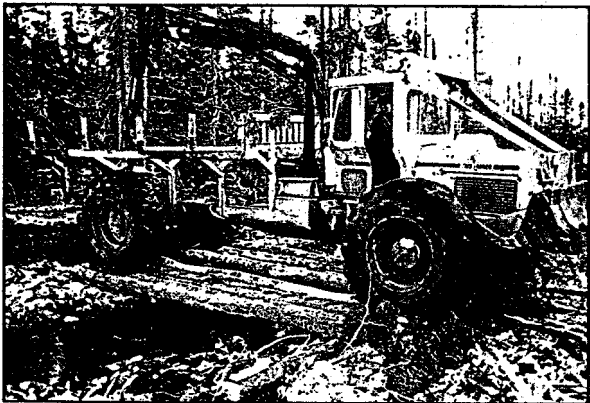
Portable bridges are economical, easy to install, and protect fish habitat.
