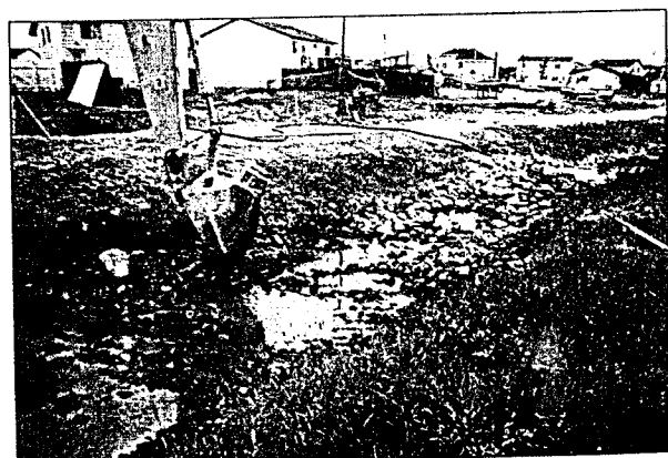
Instream excavation for stream crossing.
