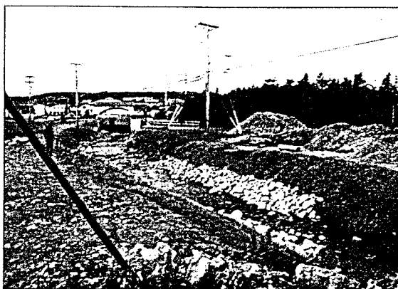
Stream crossing completed.
