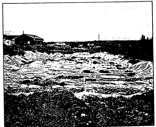
Settling basin lined with plastic.
