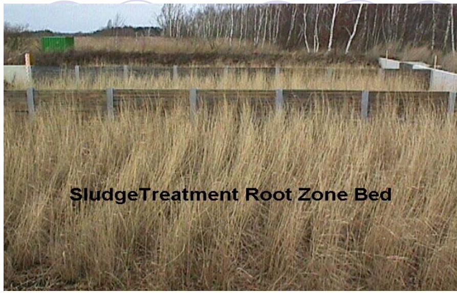
Figure 3 – Existing Sludge Treatment Beds
