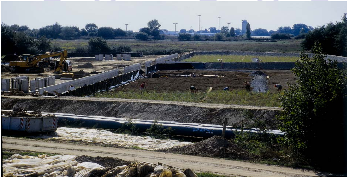
Figure 7 – Construction of a Kickuth treatment system
