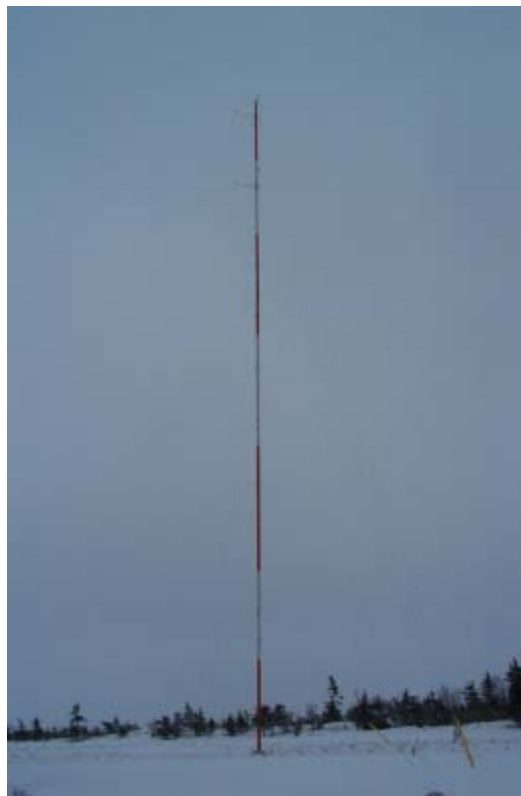
Figure 3.1 : Wind Monitoring Tower at The Arches
