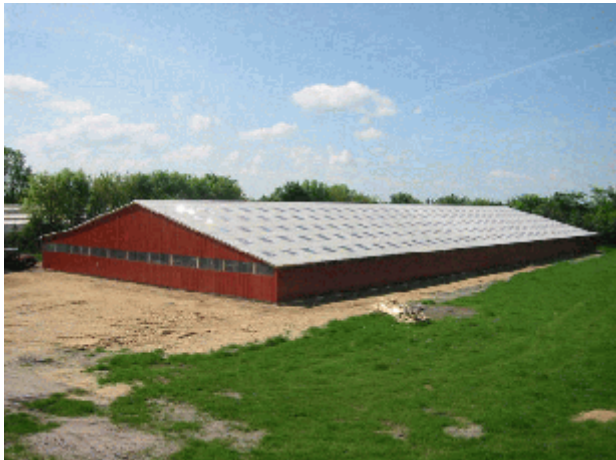
Exterior of Large Mink Shed
