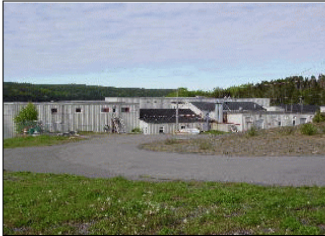
External View of Building
