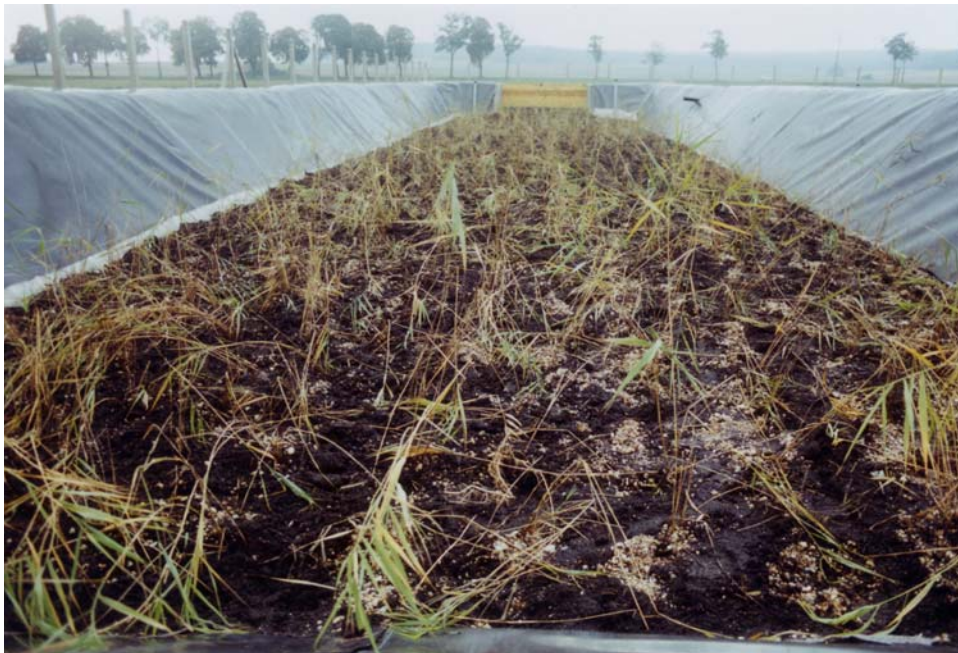
Figure 4 Typical Sludge Treatment Cell
