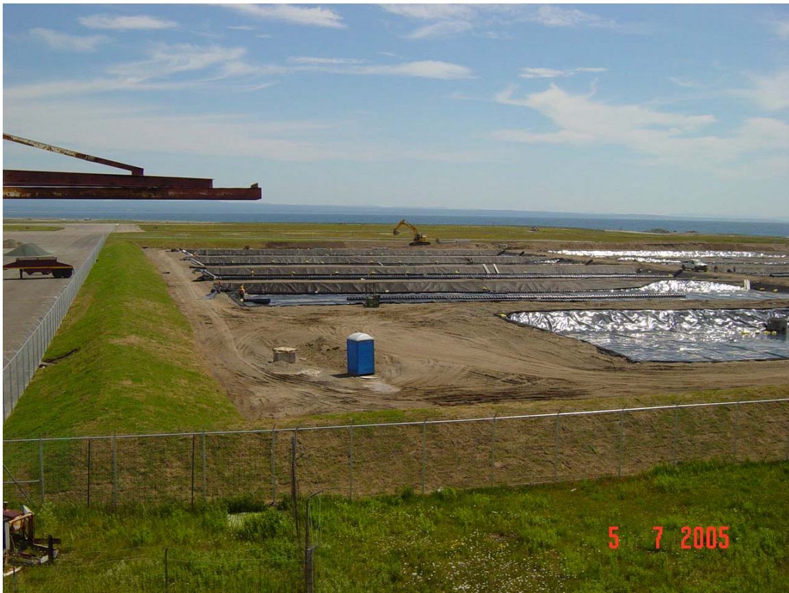
Figure 7 Construction of Main Wetland Treatment System
