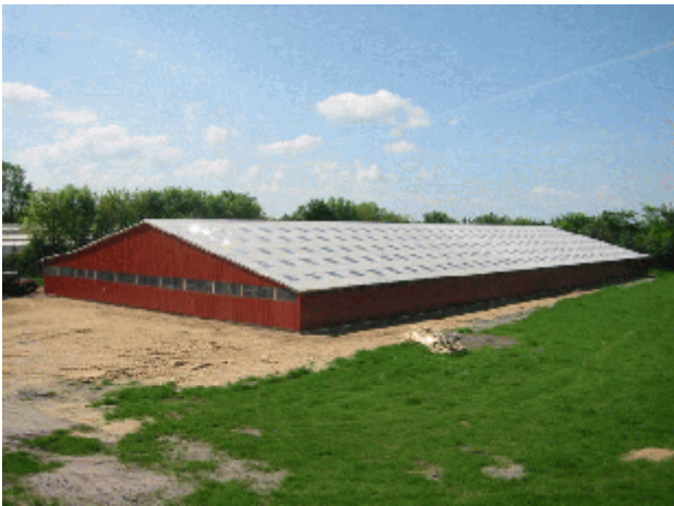
Exterior of Large Mink Shed
