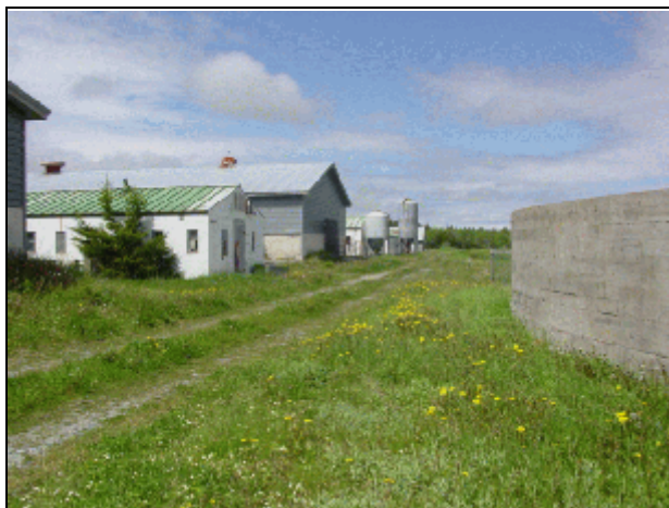
Existing Sheds and Manure Storage
