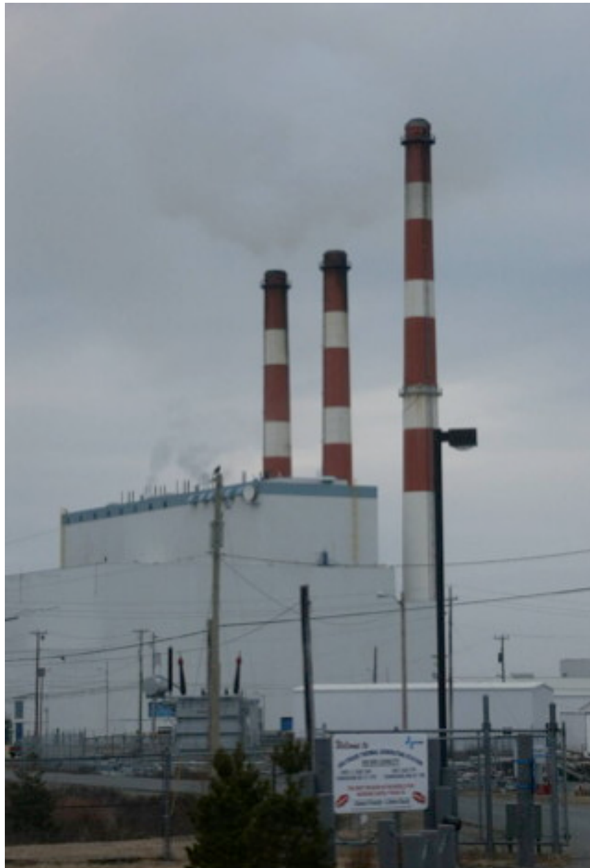
Holyrood Thermal Generation Station, 490 MW capacity
