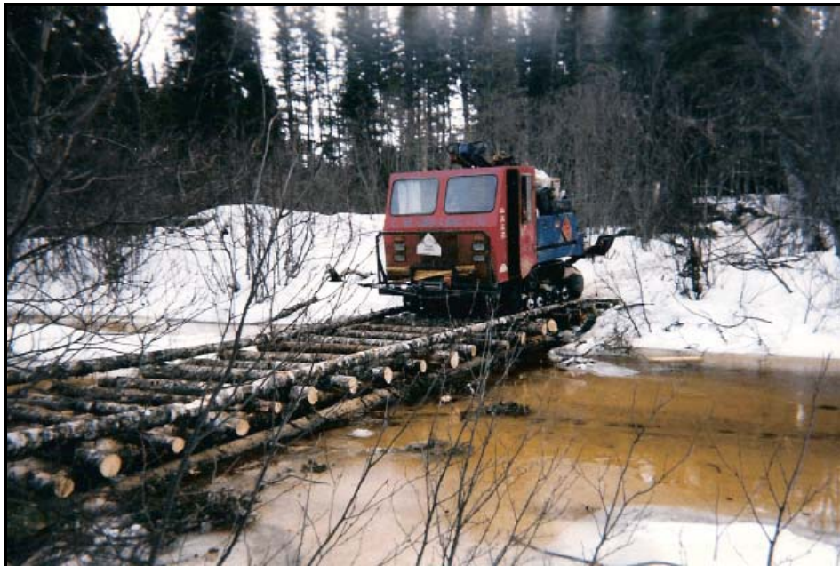
Figure 4-13 Typical Seismic Drill Rig Crossing a Temporary Bridge.
