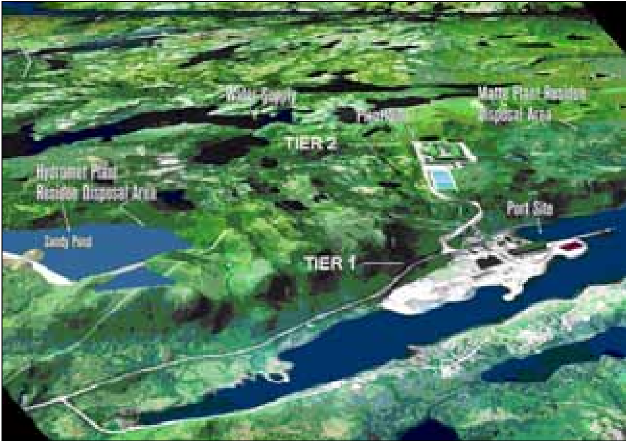
Figure 2.1 General Layout (viewed from the north)
