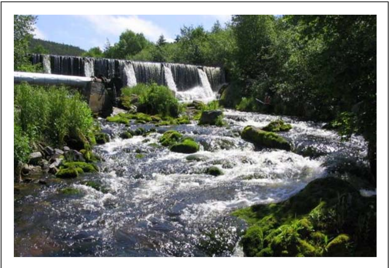
Figure 2.9 Concrete Weir Near the Mouth of Rattling Brook, June 22, 2006
