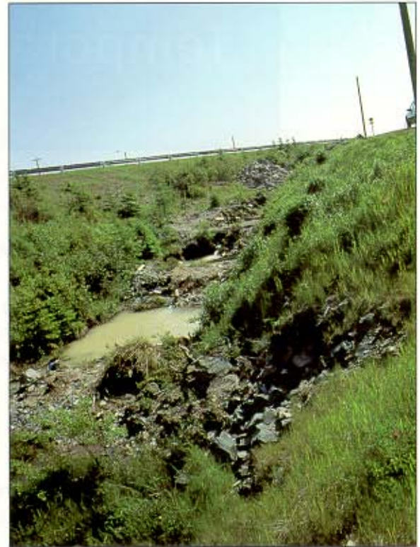
Series of rough settling basins intended for short term use.
