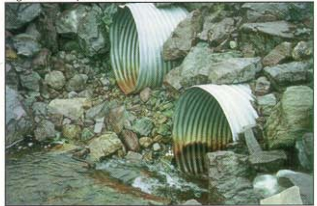
Figure 4. Multiple Culvert Installation
