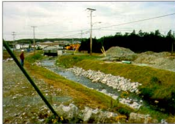
Stream crossing completed.
