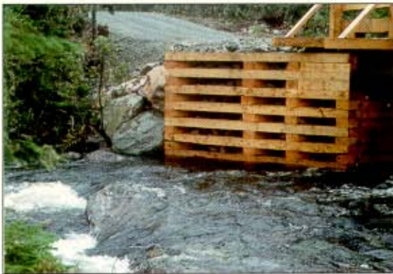
Timber crib construction: untreated/pressure treated wood.
