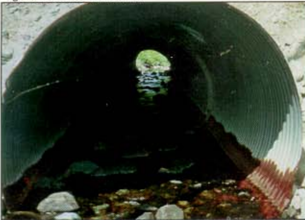
Figure 3. Countersunk Culvert
