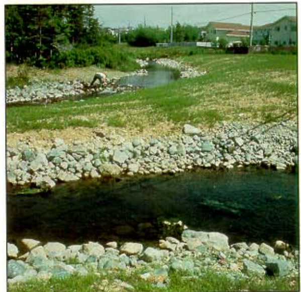
Stream bank stabilization using rip rap and hydroseed.
