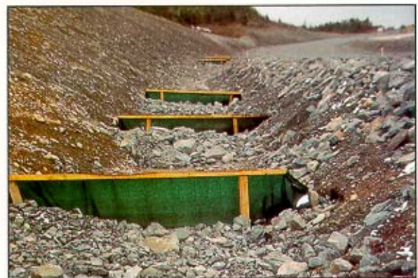
Filter fabric used for low point protection.
