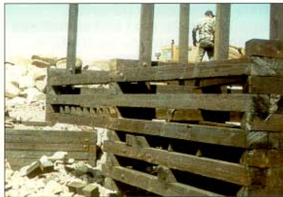
Timber crib construction for marine environment.
