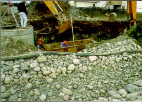
Stream bed restored.
