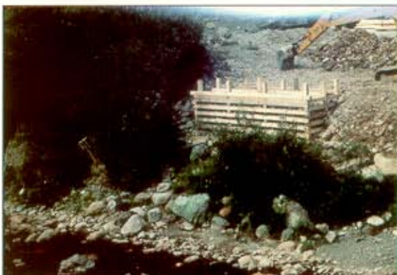
Bridge abutments outside wetted stream perimeter.
