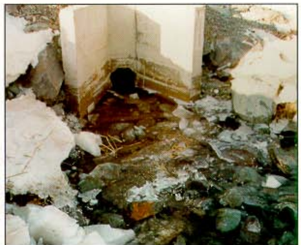
Storm drain outlet channel - stabilization.
