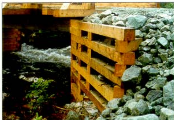
Infill materials for timber cribs.
