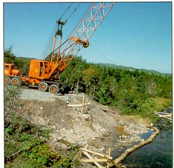
Cofferdam isolating stream margin work area from stream flow.
