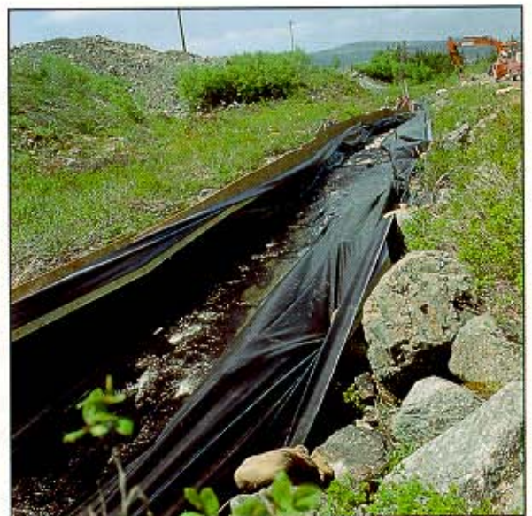
Temporary diversion - channel liner.
