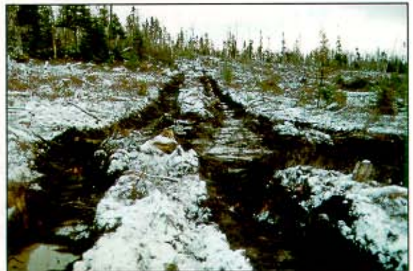
Mudlogs deflect water off the forwarder trail and onto the forest floor.
