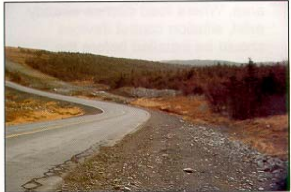
Highway low point (centre).
