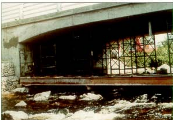
"False Work" to support concrete bridge decking.
