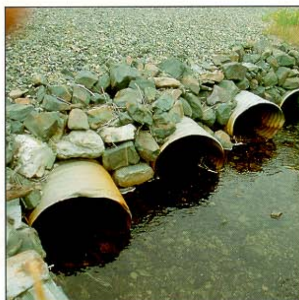
Stabilization of culvert outlets - rip rap.
