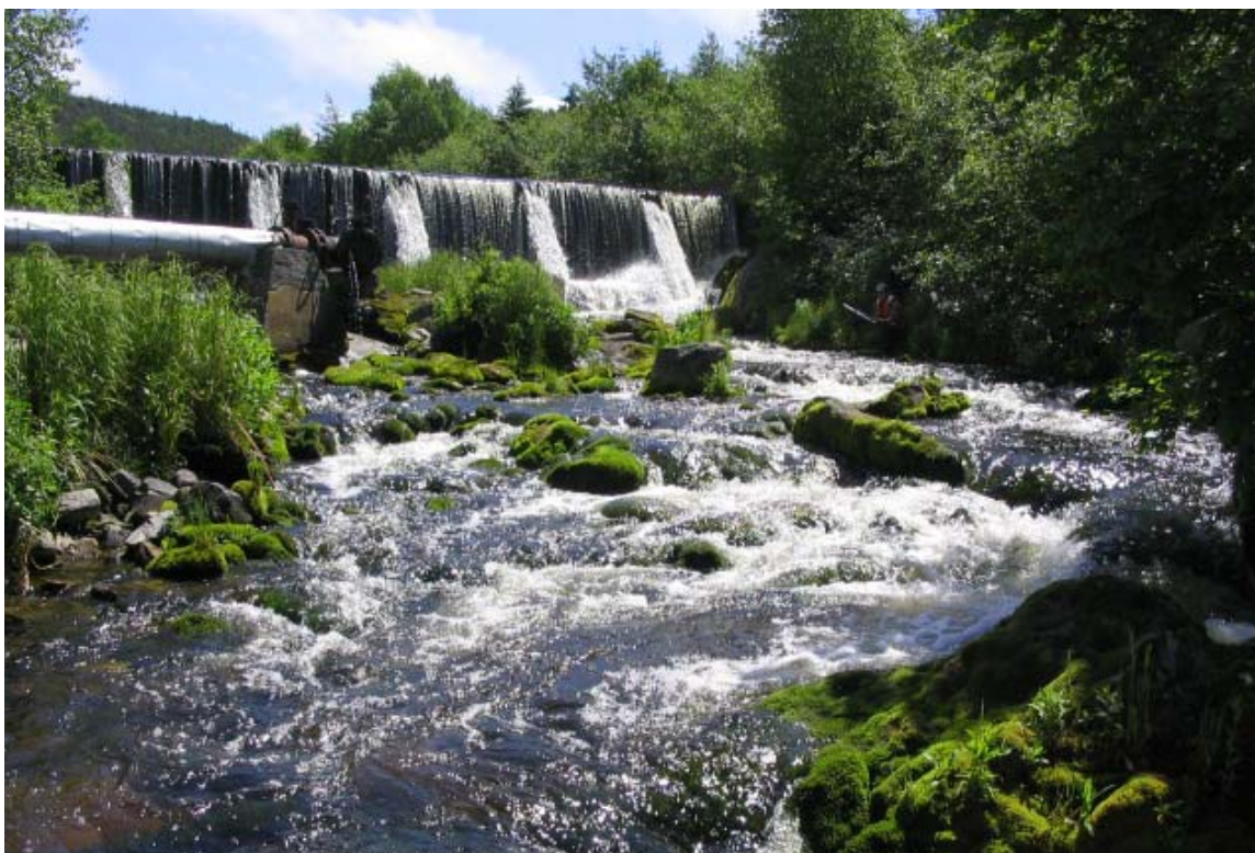
Figure 9.3 Concrete weir near the mouth of Rattling Brook, June 22, 2006.
