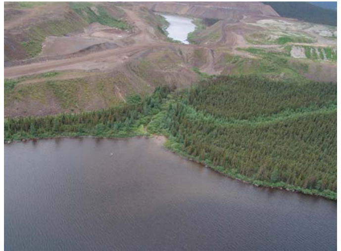
28 Downstream of Culvert 6A
