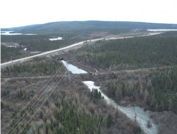
29 Culverts at 6B
