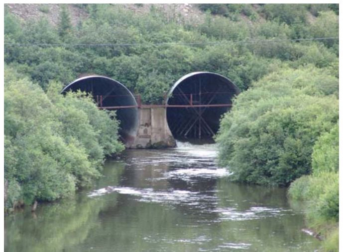
30 Culverts at 6B
