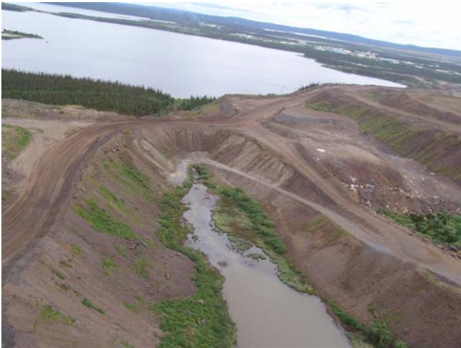
27 Inlet of Culvert 6A
