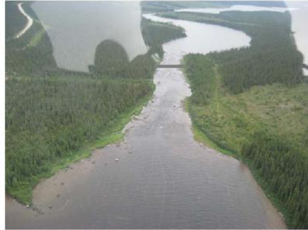
2 Canning Narrows Looking Downstream
