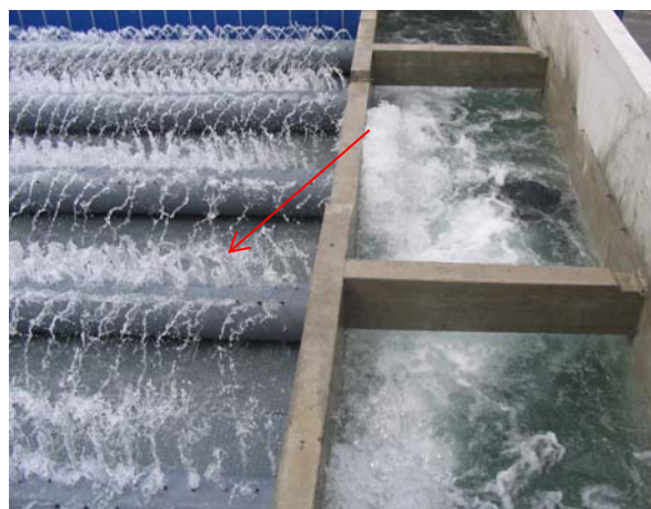
Picture 20 Example of perforated pipes red arrow
