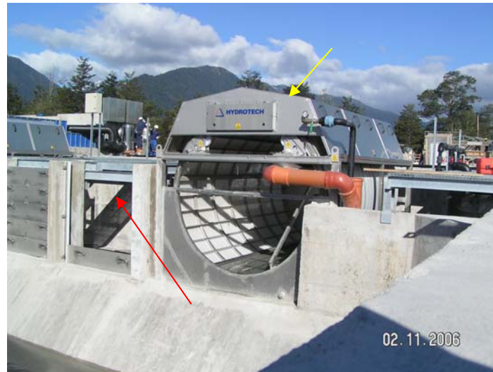
Picture 10 Example of a bypass (red arrow ) Manometer for pressure control (yellow arrow)
