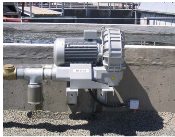
Picture 18 Blower for the moving bed filter which keeps the bio media in motion
