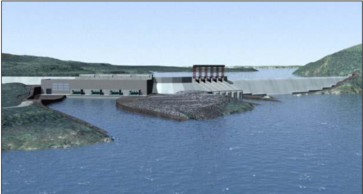
Figure 6-1 Muskrat Falls Generating Facility
