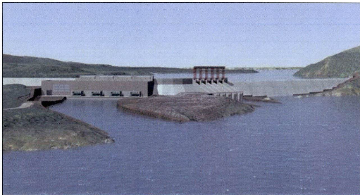
Figure 6-1 Muskrat Falls Generating Facility
