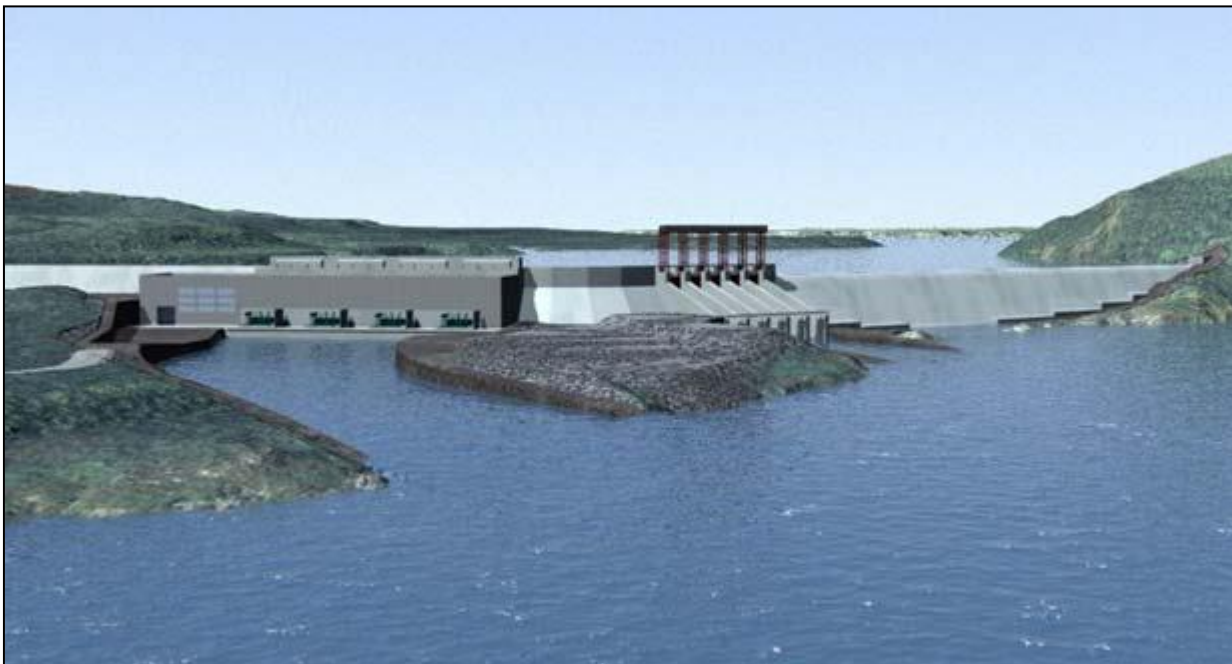
Figure 6-1 Muskrat Falls Generating Facility
