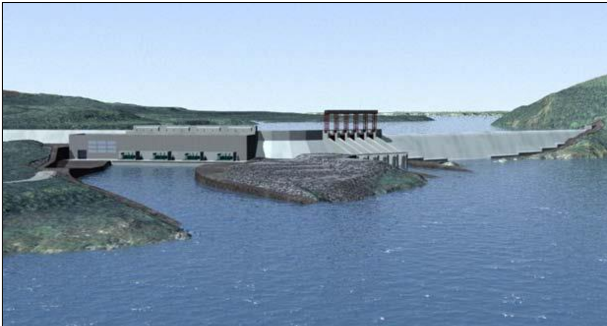
Figure 6-1 Muskrat Falls Generating Facility
