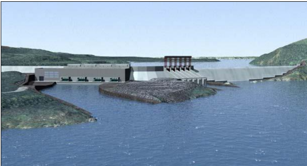
Figure 11-1 Muskrat Falls Generating Facility
