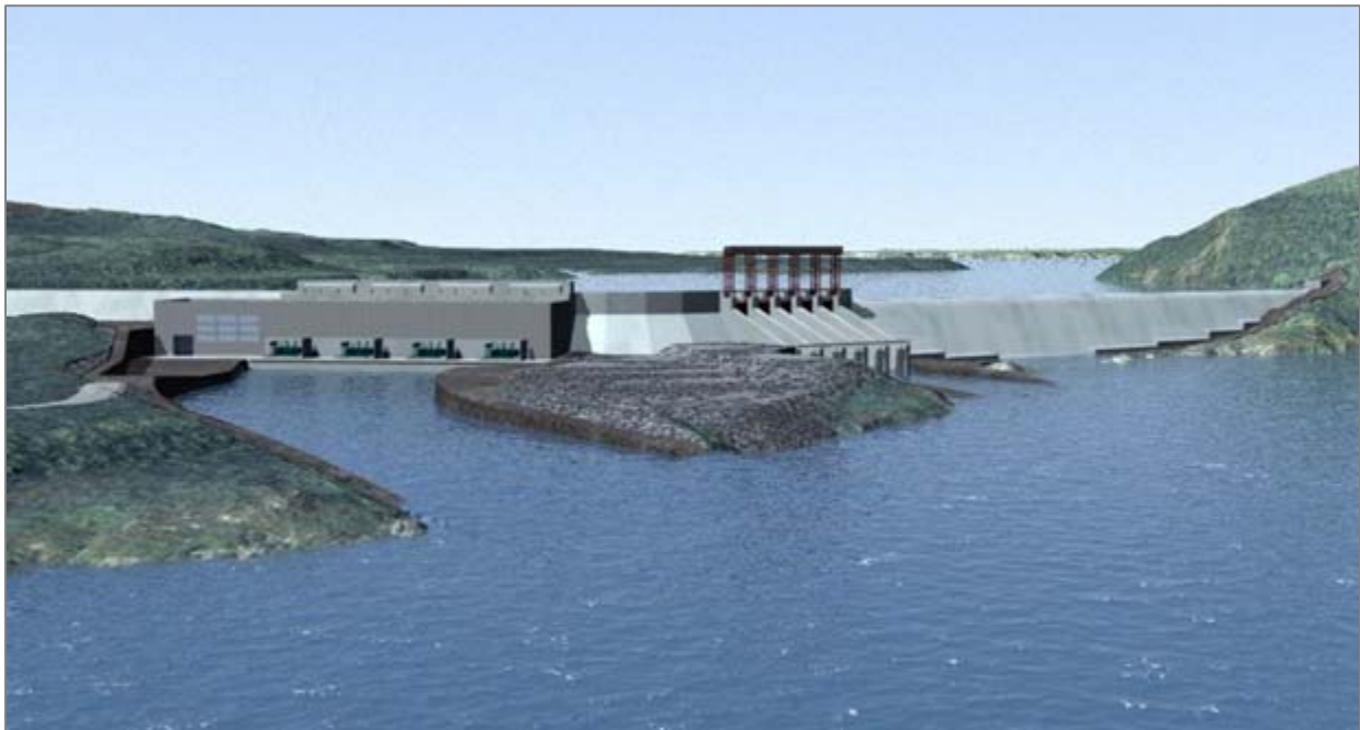
Figure 2-1: Muskrat Falls Generating Facility (Component 1)
