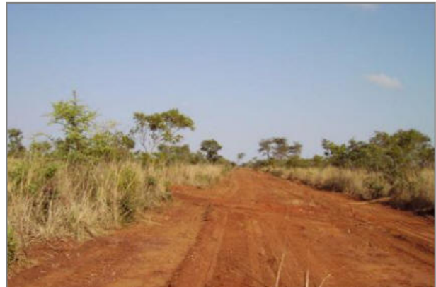
Figure 5-14: Example of grubbed and cleared path
