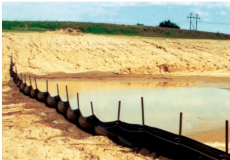
Figure 5-33: A well constructed silt fence
