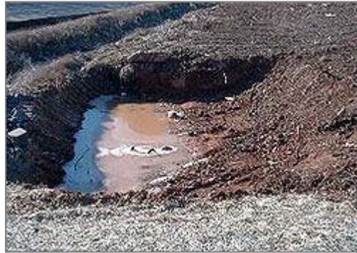
Figure 5-39: Sediment Trap
