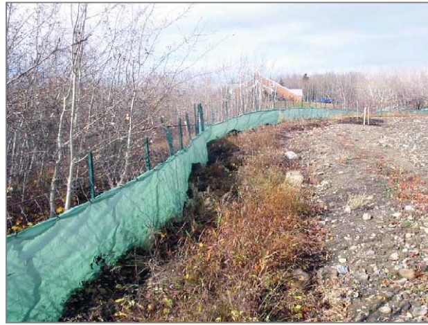
Figure 5-9: Tarp fence outlining a vegetation buffer zone
