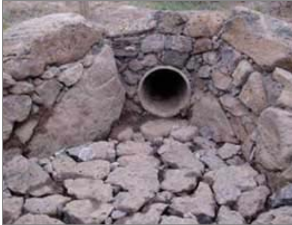
Figure 5-31: Correct Construction of Rock Energy Dissipaters
