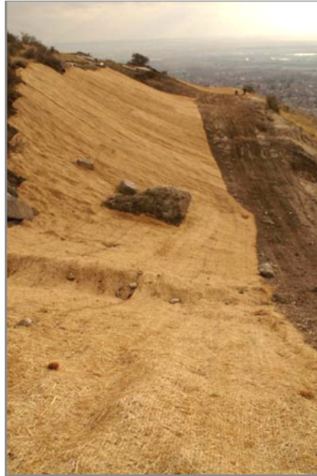
Figure 5-24: Photograph of Erosion Control Blanket used on a slope
