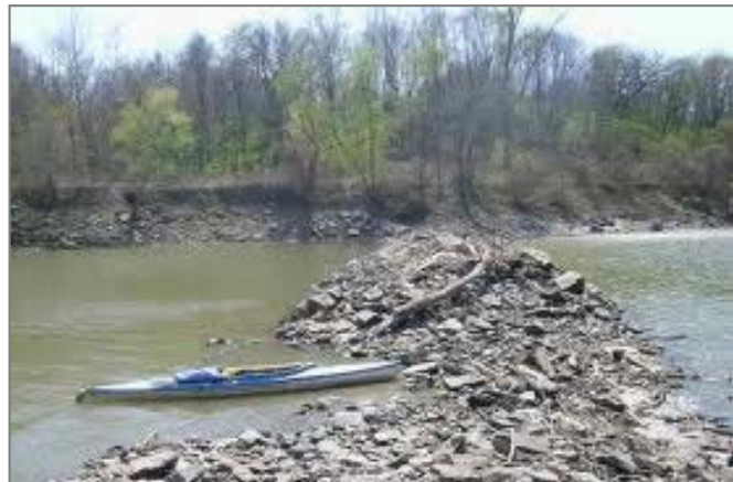
Figure 5-30: Photograph of a Rock Constructed Dike
