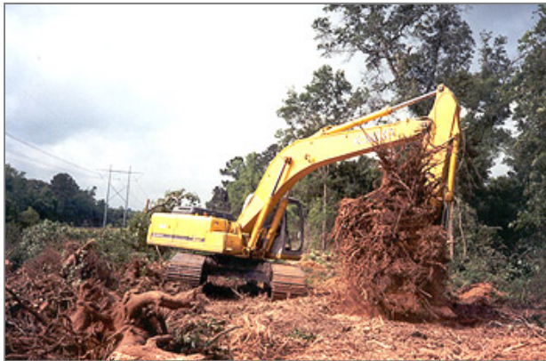
Figure 5-13: Example of grubbing activities
