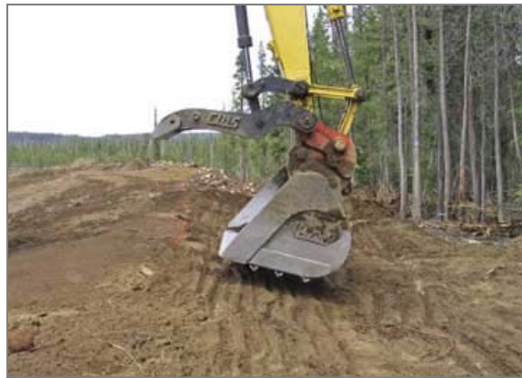
Figure 5-21: Photograph of grooving slope treatment method
