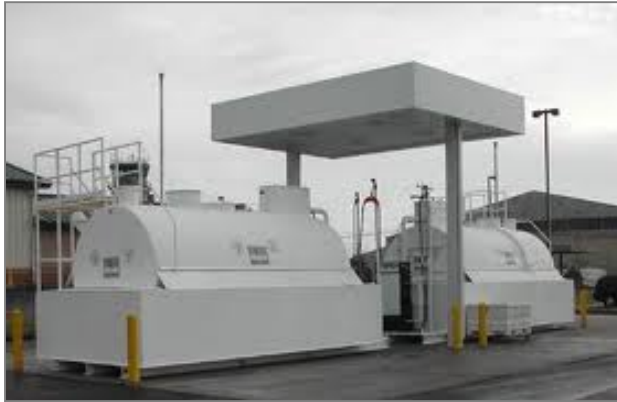
Figure 5-5: Acceptable fuel storage with dykes
