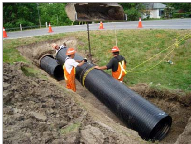
Figure 5-8: Example of culvert installation
