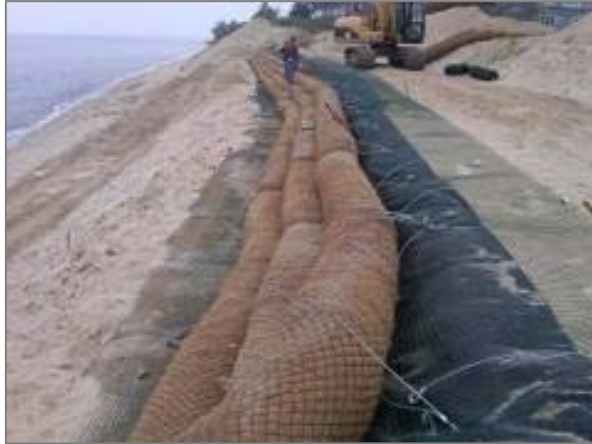
Figure 5-25: Photograph of Fibre Rolls used to stabilize
