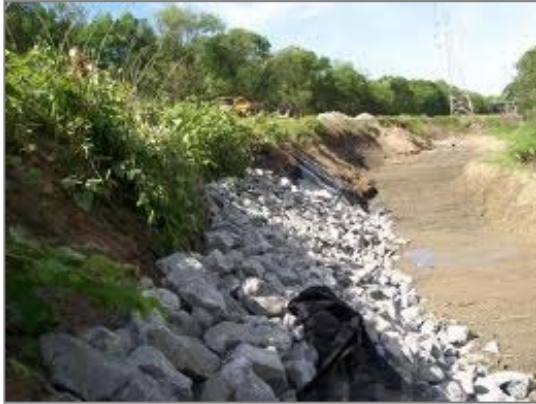
Figure 5-27: Photograph of Rip Rap placed along a slope
