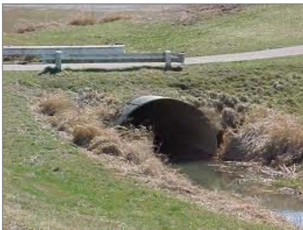
Figure 5-7: Example of well installed culvert
