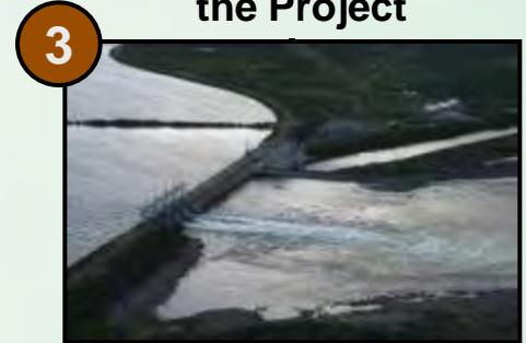
Menihek Dam - 35km from the Project
