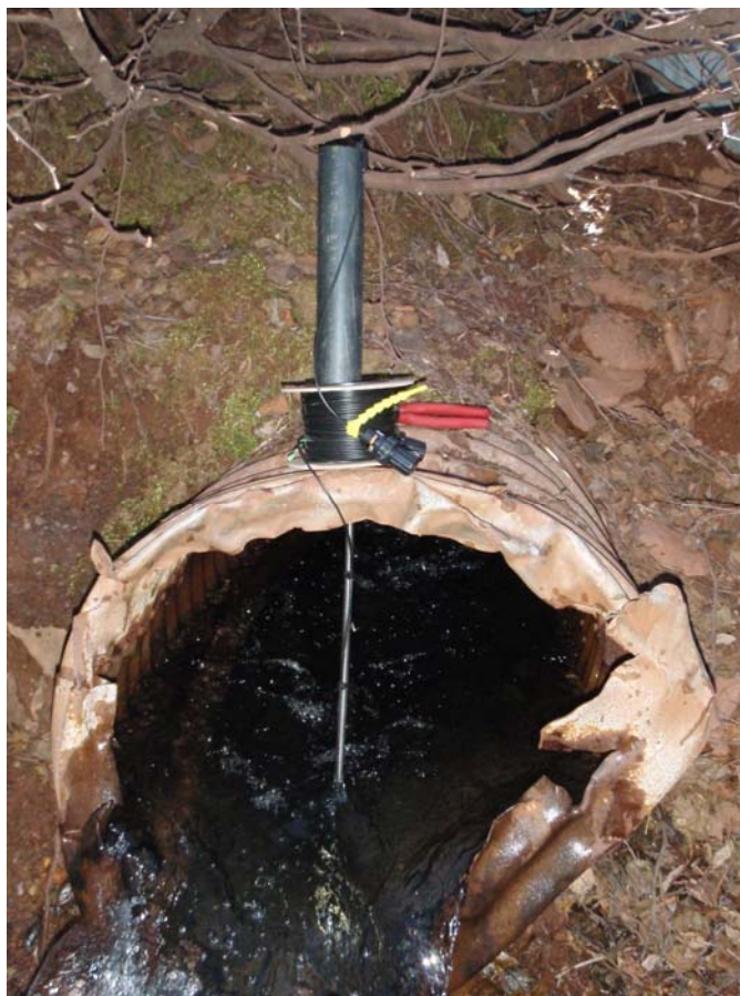
Photograph 3: SG4 Levelogger Looking West
