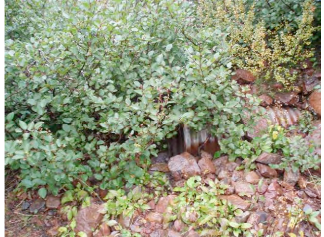
RLC-17 (view looking upstream)
