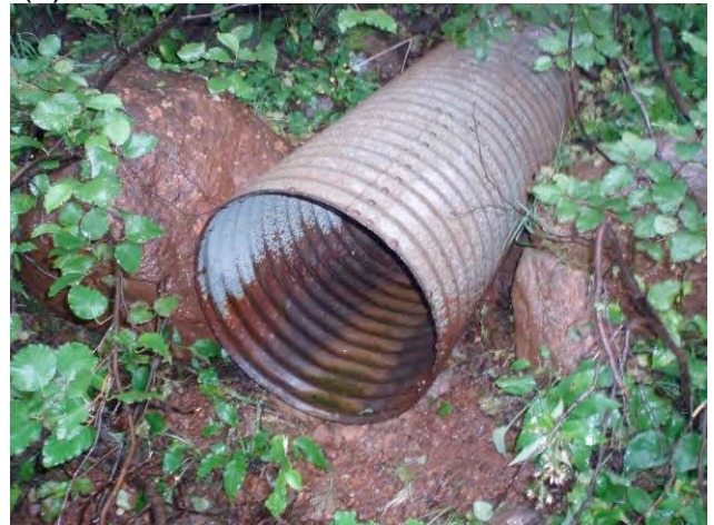
RLC 17 (view from downstream)
