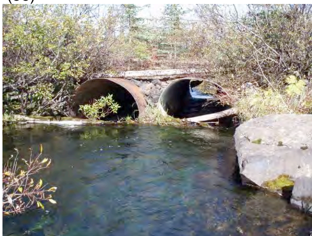
AR-1 Upstream-3 (view looking upstream)
