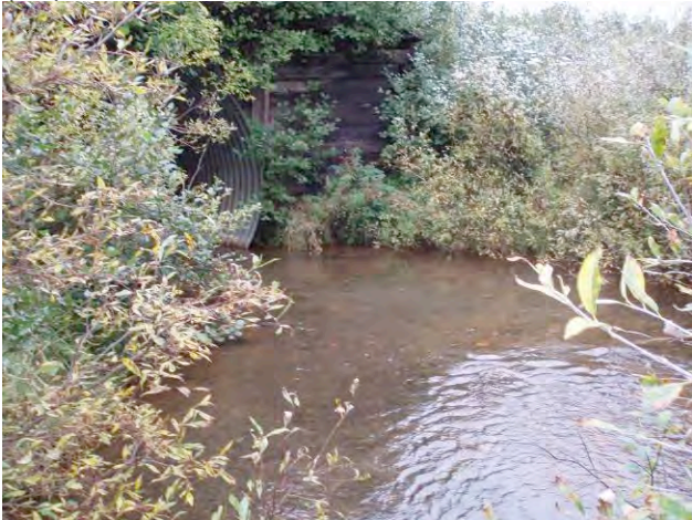
RLC-27a (view looking downstream)
