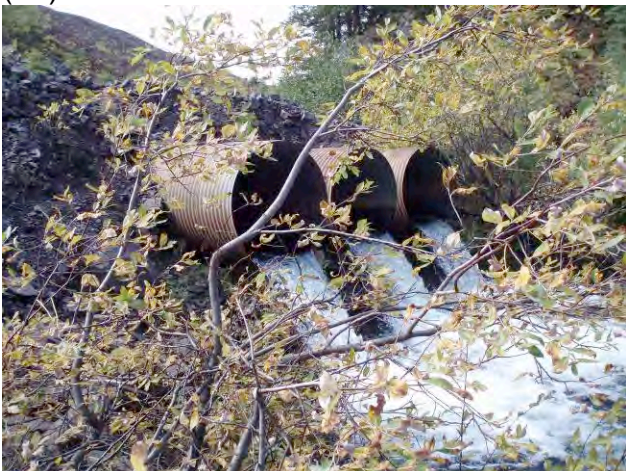
AR-1 (view from downstream)
