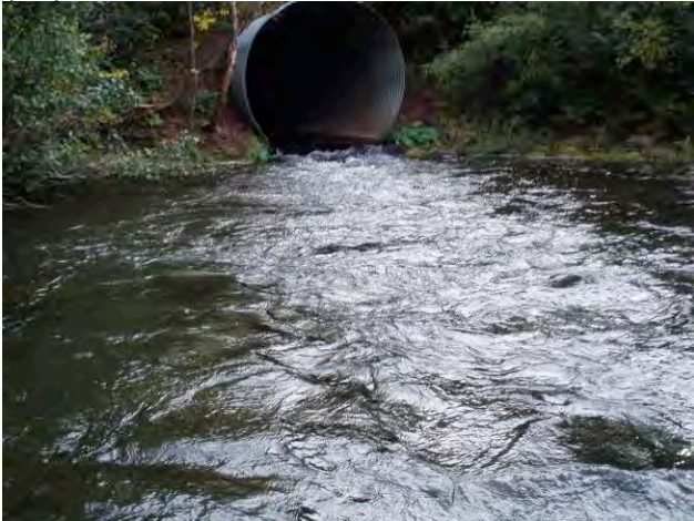
RLC-26 (view from downstream)
