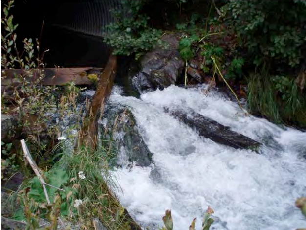
RLC-27 (view from downstream)
