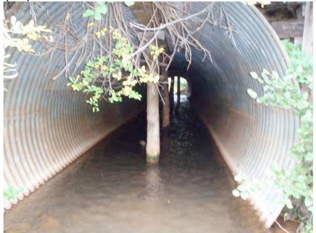
RLC-27a (view from upstream)
