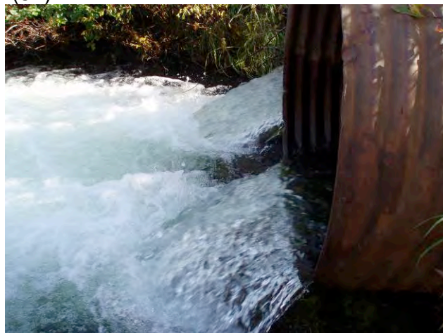
AR-1 Upstream-3 (view looking downstream)
