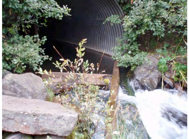
RLC-27 (view from downstream)
