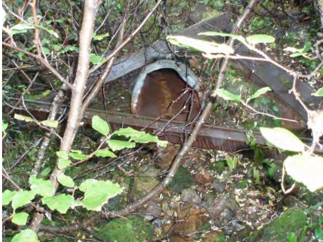
RLC-3a (view from upstream)
