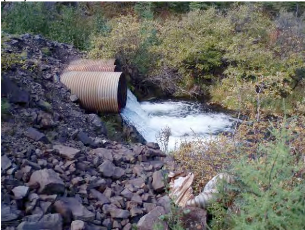
AR-1 (view from downstream)
