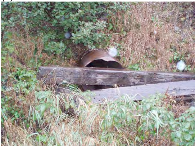
RLC-3a (view from downstream)
