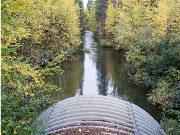
RLC-26 (view looking upstream)
