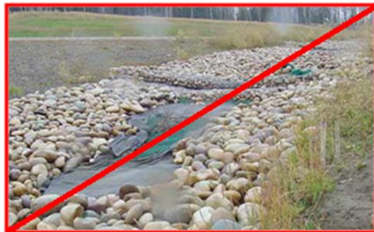
Figure 11-28 - Photograph of failed Rip Rap Protection a Slope
