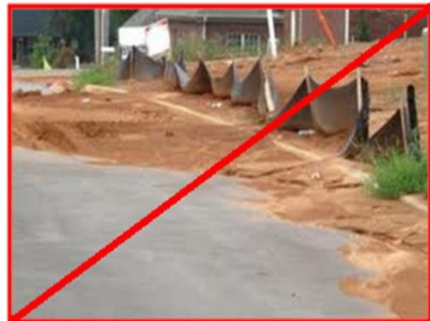
Figure 11-37 - Examples of Poorly Installed Silt Fences
