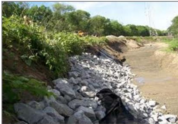
Figure 11-27 - Photograph of Rip Rap Placed Along a Slope
