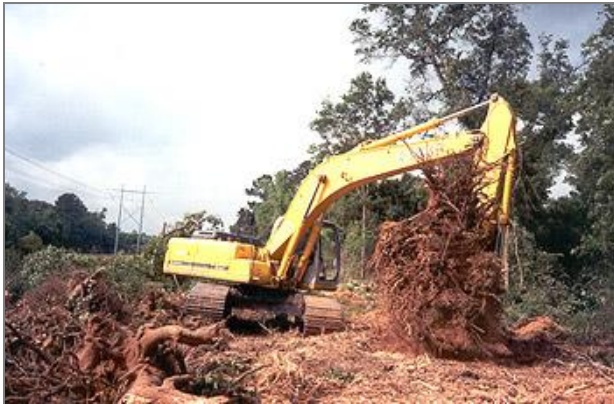
Figure 11-13 - Example of Grubbing Activities
