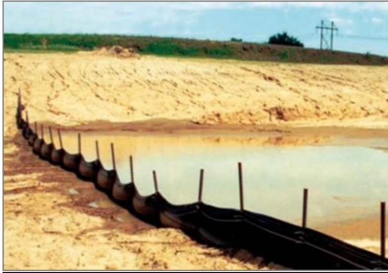
Figure 11-33 - A Well Constructed Silt Fence
