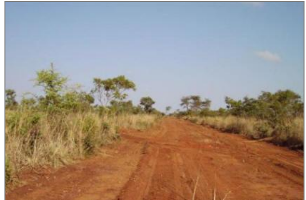
Figure 11-14 - Example of Grubbed and Cleared Path
