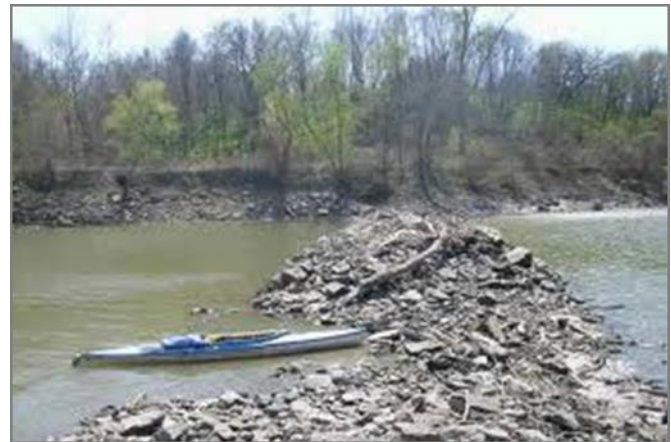
Figure 11-30 - Photograph of a Rock Constructed Dike
