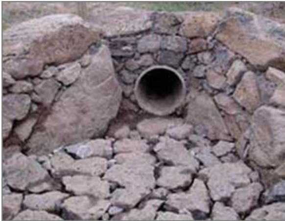
Figure 11-31 - Correct Construction of Rock Energy Dissipaters
