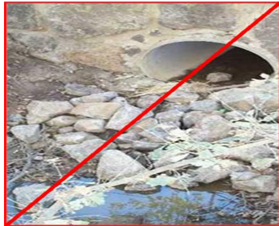
Figure 11-32 - Incorrect Construction of Rock Energy Dissipaters
