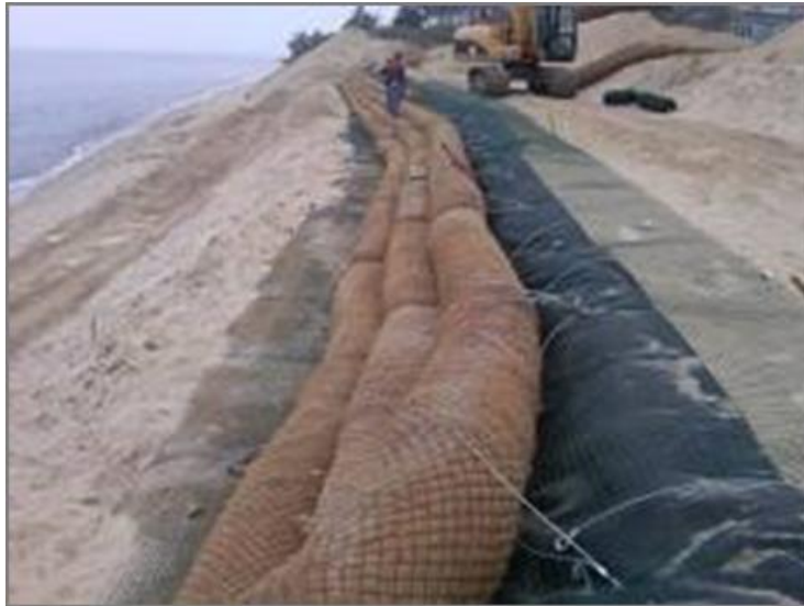
Figure 11-25 - Photograph of Fibre Rolls used to Stabilize
