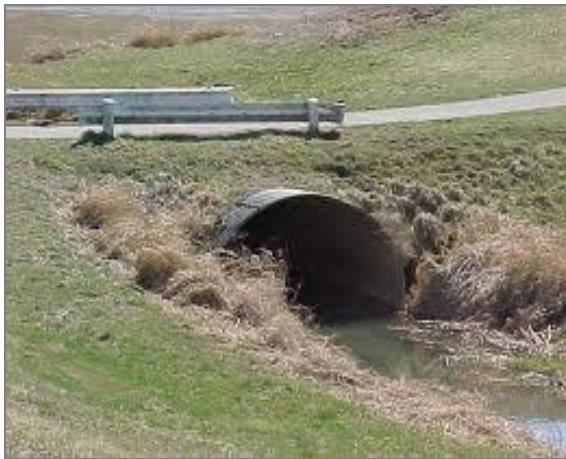
Figure 11-8 - Example of Well Installed Culvert
