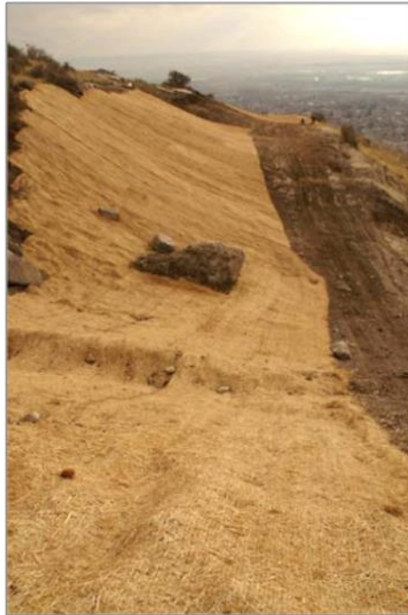
Figure 11-24 - Photograph of Erosion Control Blanket used on a Slope
