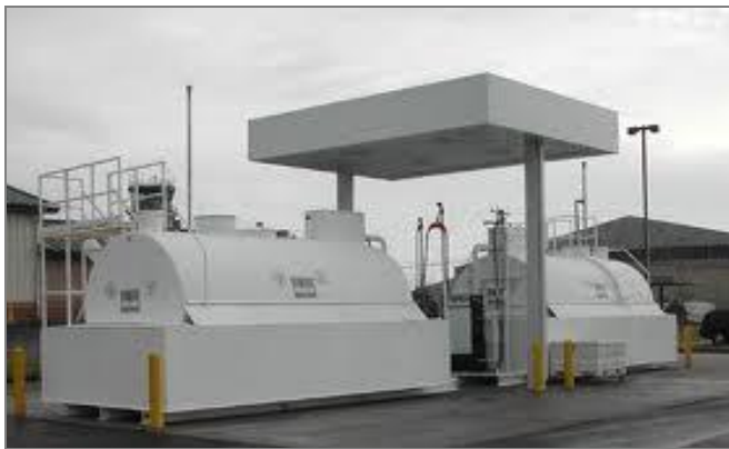
Figure 11-6 - Acceptable Fuel Storage with Dykes
