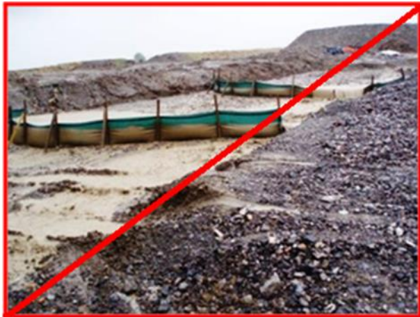
Figure 11-36 - Examples of Poorly Installed Silt Fences
