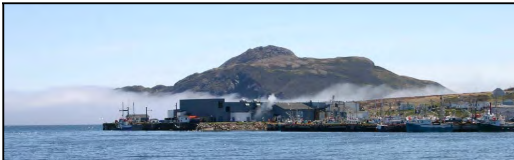
Figure 7-2: St. Lawrence Harbour, NL. (Photo courtesy of N. Wilson)
