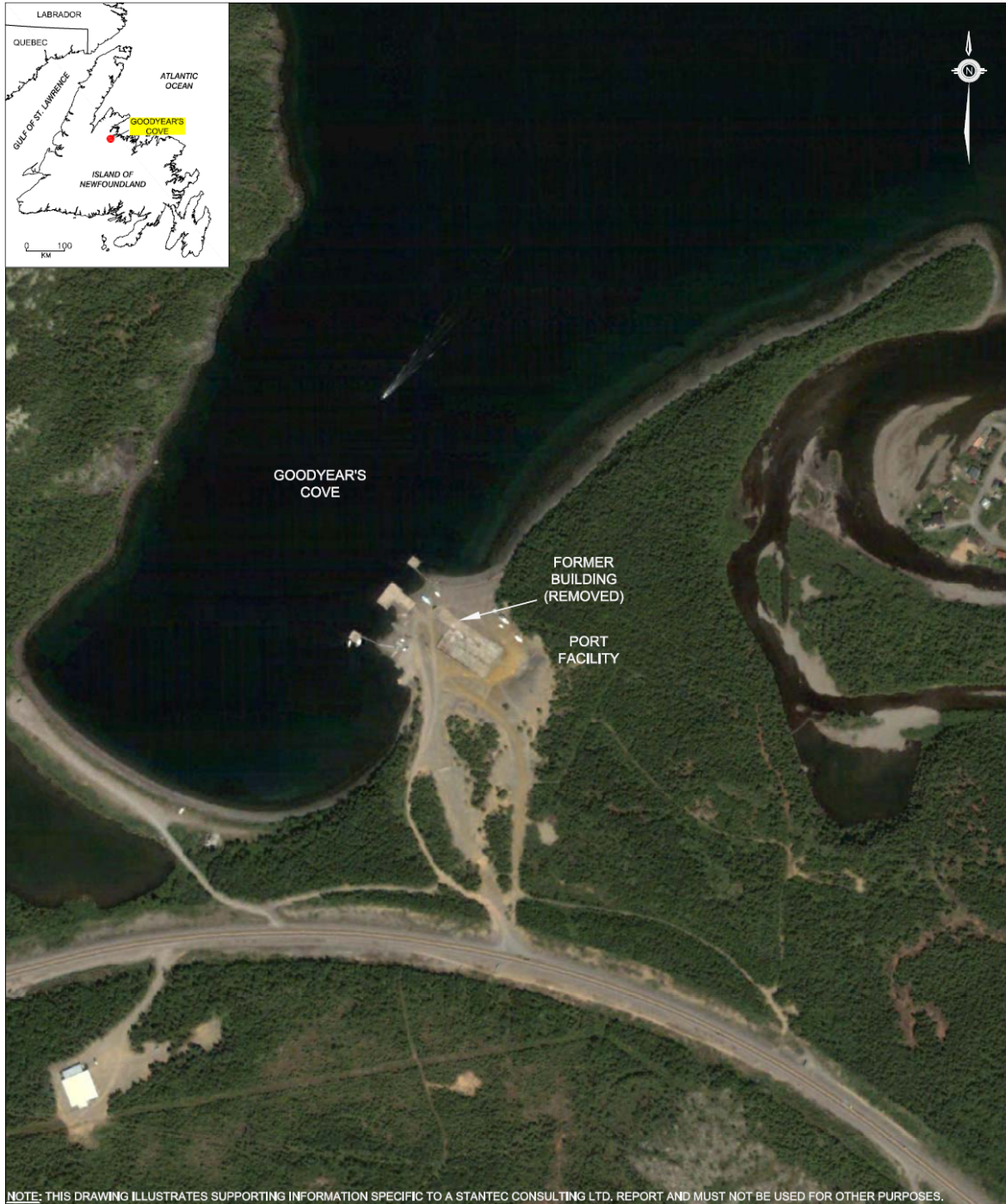
Figure 2-7 Aerial Photo of the Goodyear's Cove Port Site
