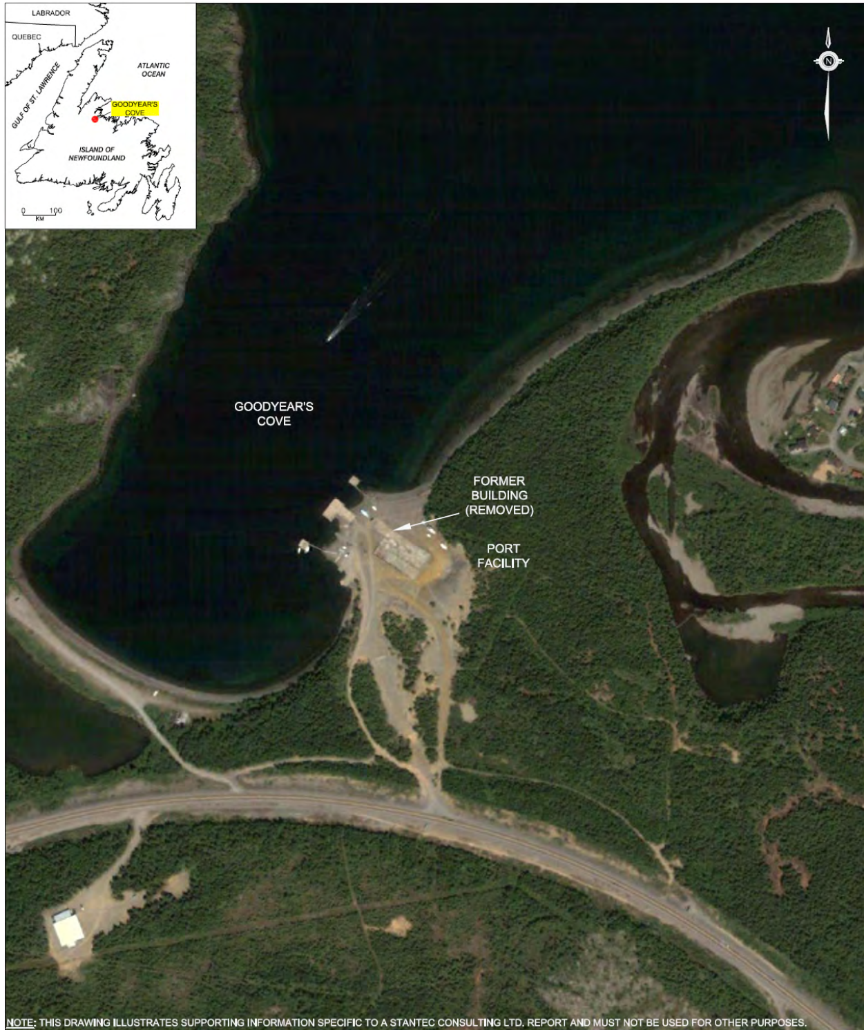
Figure 3-18 Aerial Photo of the Goodyear's Cove Port Site`
