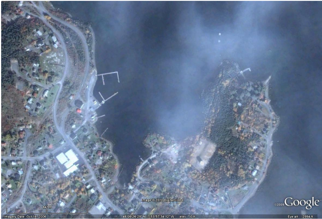
Overview of Dark Hole and existing Clarenville Marina.
