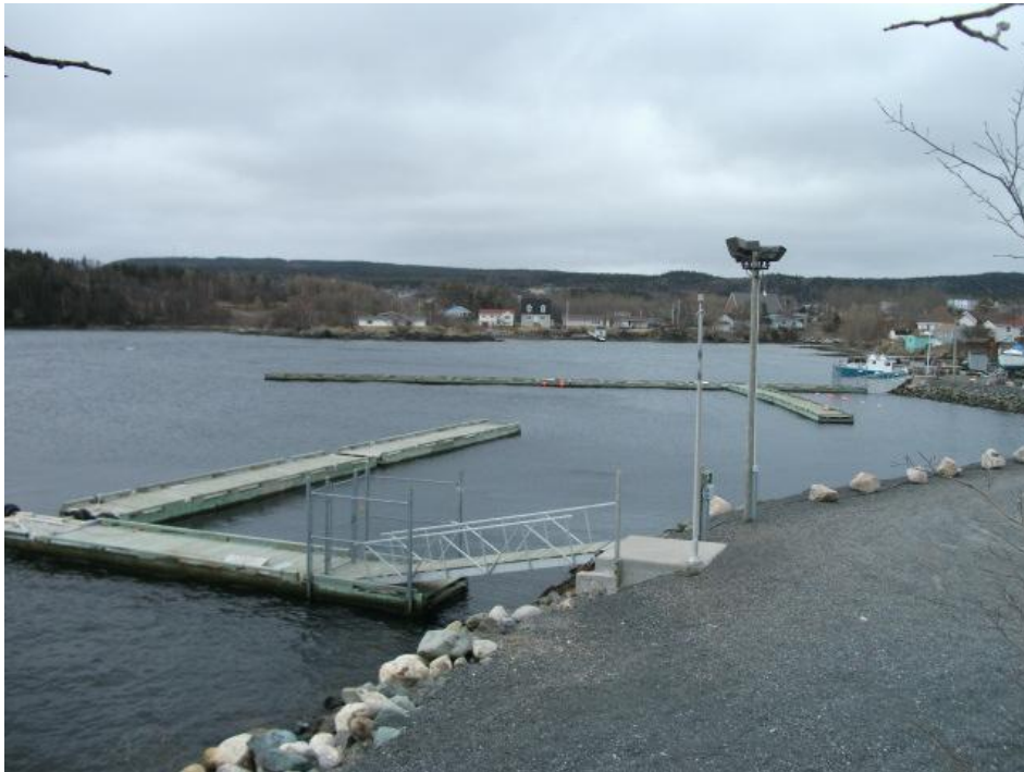
Photo No. 3: “North” dock in foreground; “South” dock in background.
