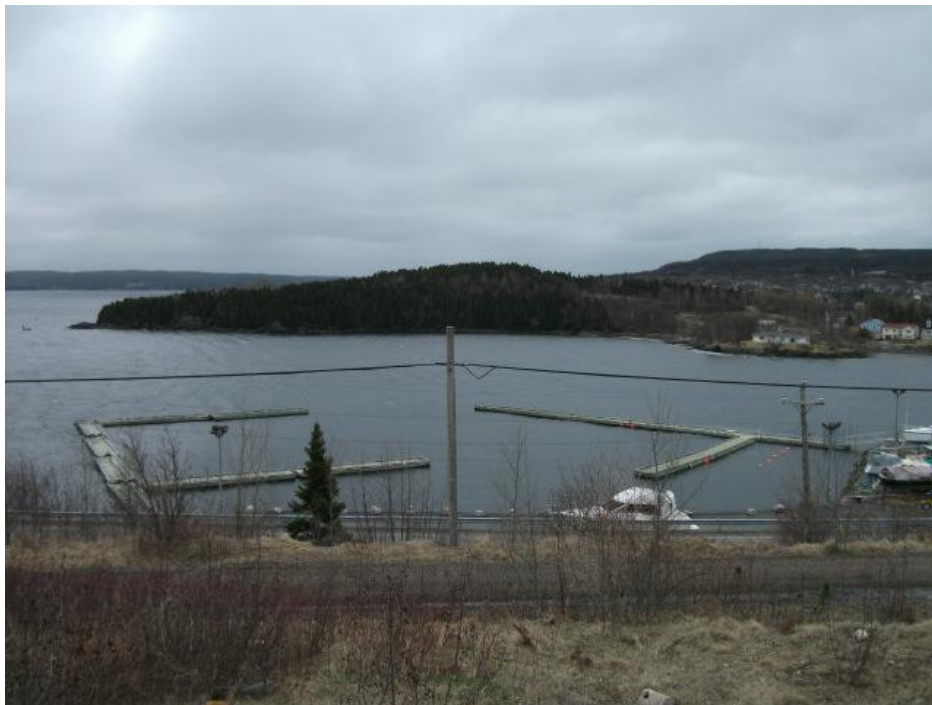
Photo No. 1: Overview of existing marina.
