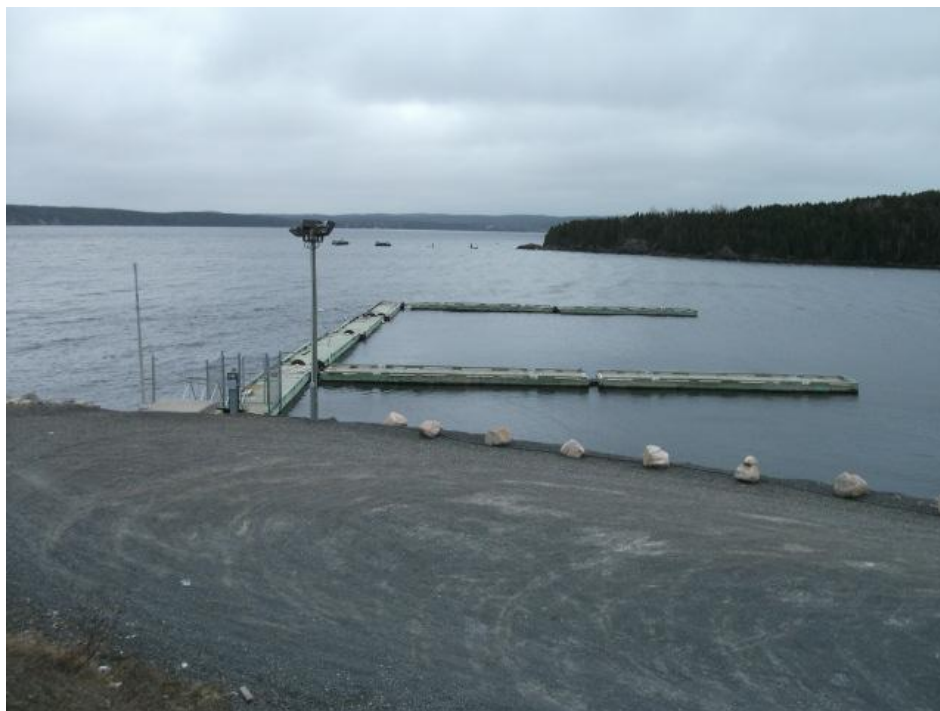
Photo No. 2: "North" dock.
