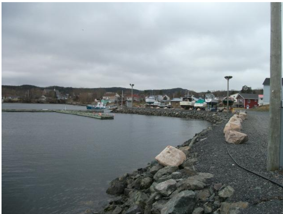
Photo No. 6: Partial view of "South" dock and original rock infilling of cove.
