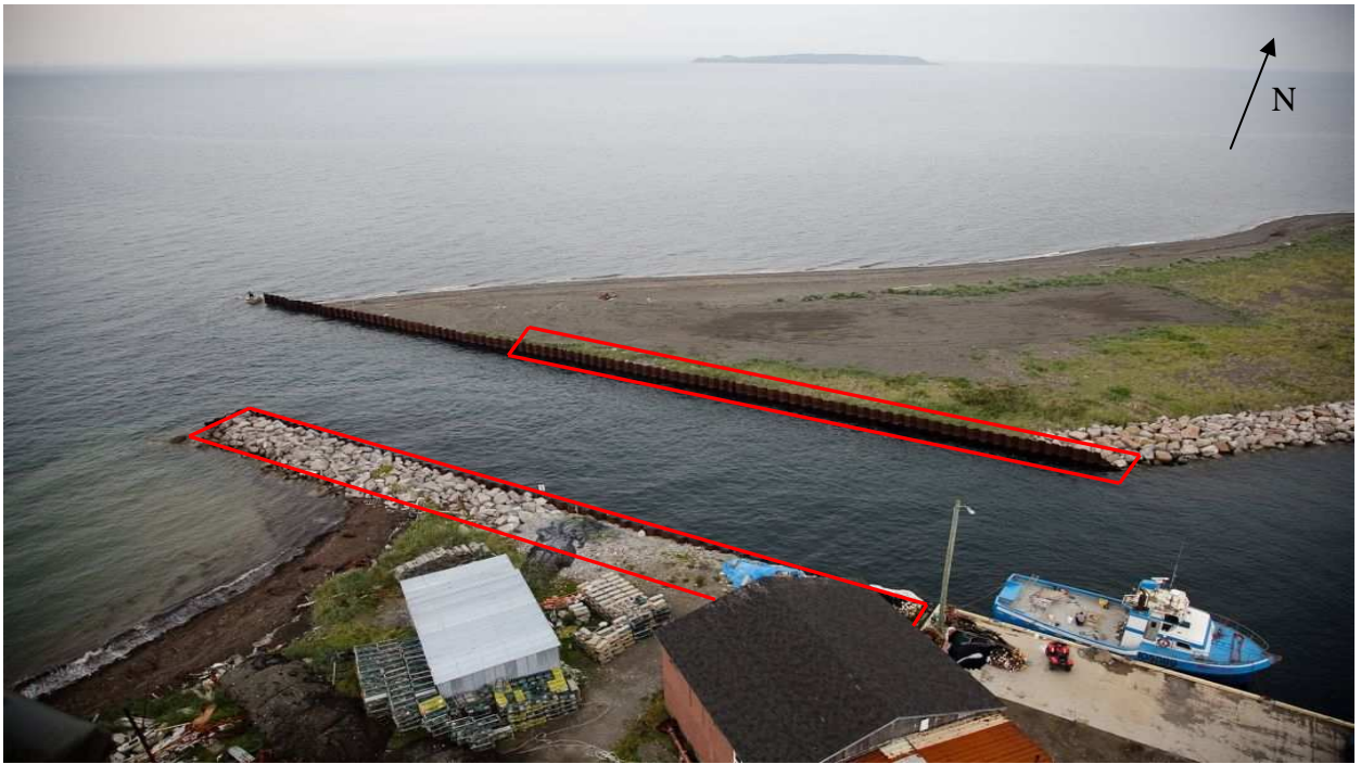
Appendix A-5. Future phases: Training wall removal (north and south side).
