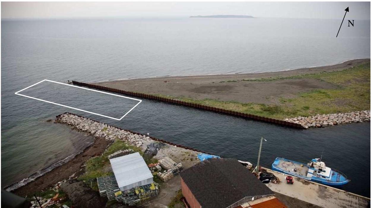
Appendix A-4. Phase 1: Channel dredging
