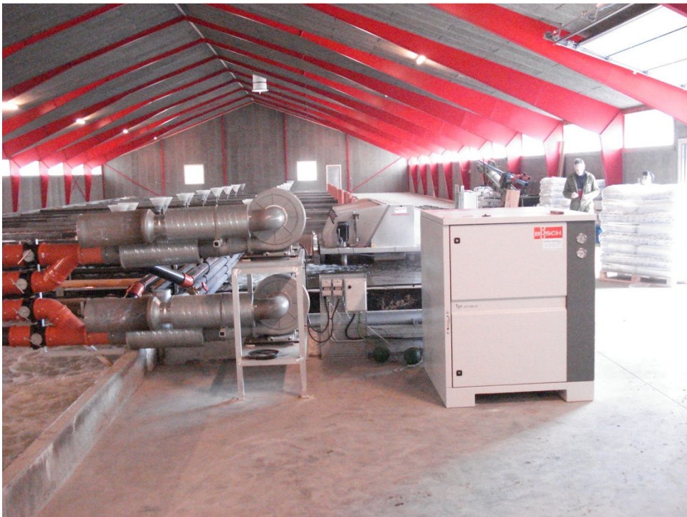
Capsel and Ventur blowers for aeration and degassing capacity up to 1.500 m 3 /hour each
