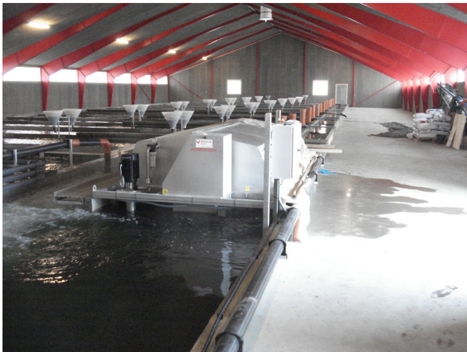
Hydrotech microscreen with 40 \mu screen
