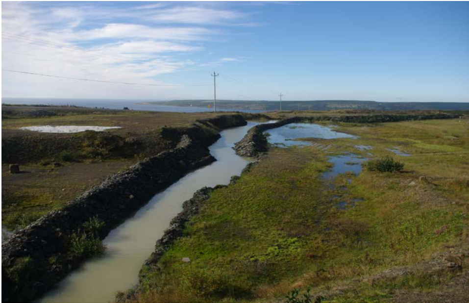
Figure 6 Drainage Ditches and Berms Southwest of the Landfill
