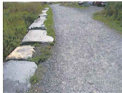
Stone edging used to retain a walk surface.
