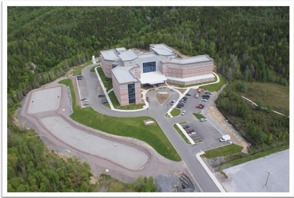
Figure 17: Corner Brook LTC Facility featuring two Abydoz Engineered Wetlands for Sewage Treatment (Prior to Plant Establishment).
