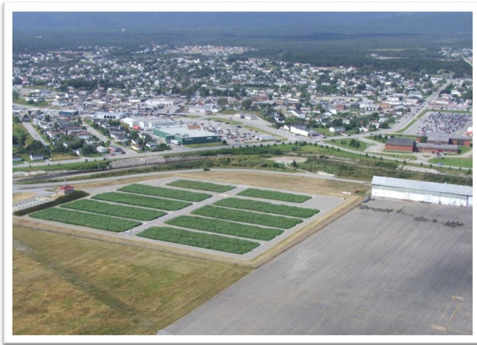
Figure 13: Stephenville Engineered Wetland System
