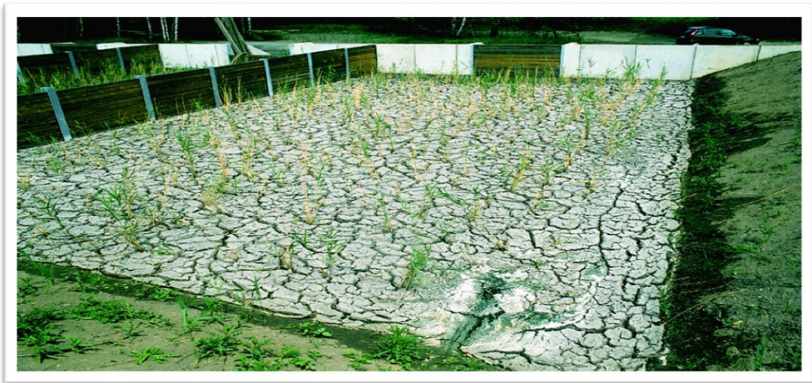
Figure 12: Abydoz Engineered Wetland Sludge Treatment Cell ready for removal.
