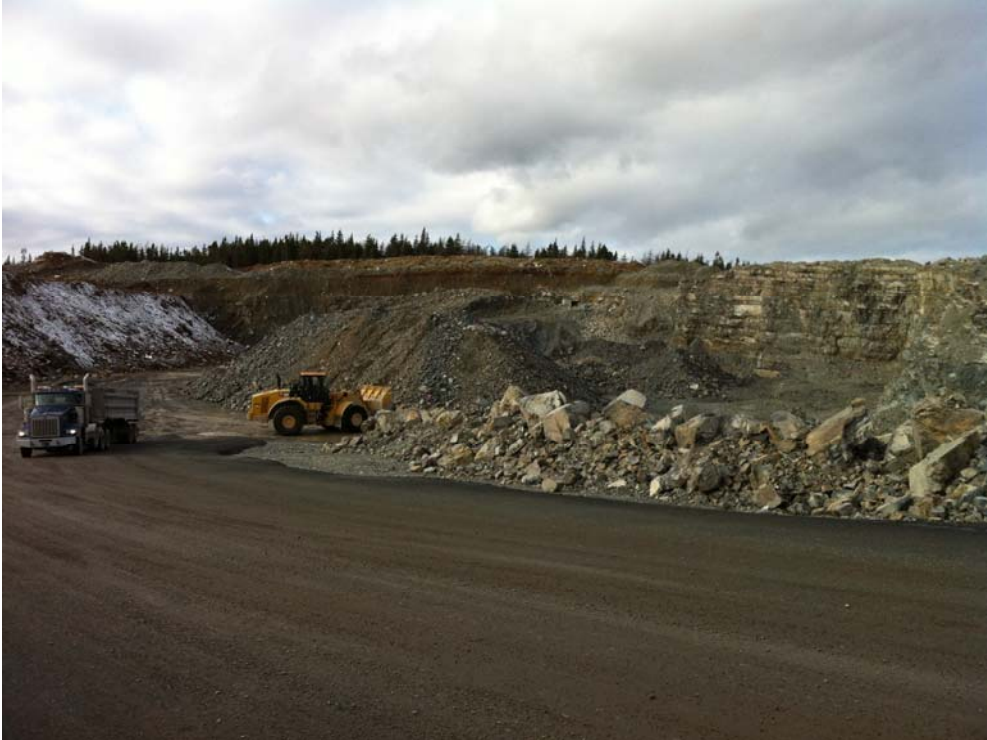
Figure 4: Active quarry operation, ~1.5 km north of the proposed Gear Pond alternative aggregate source area.
