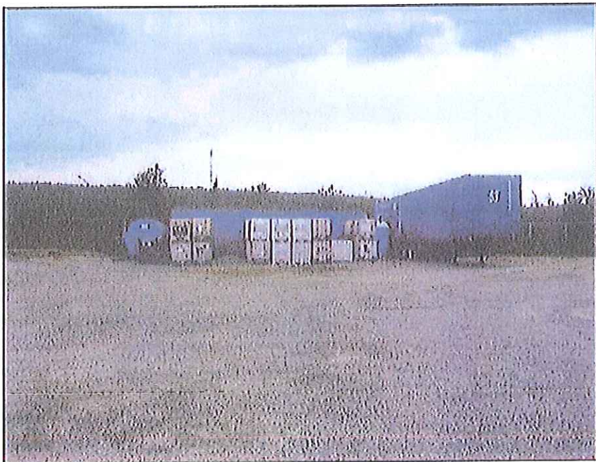
Plastic tote storage area, new drum storage trailers (behind totes), 22,730 L AST (left) and transport trailer looking northeast.
