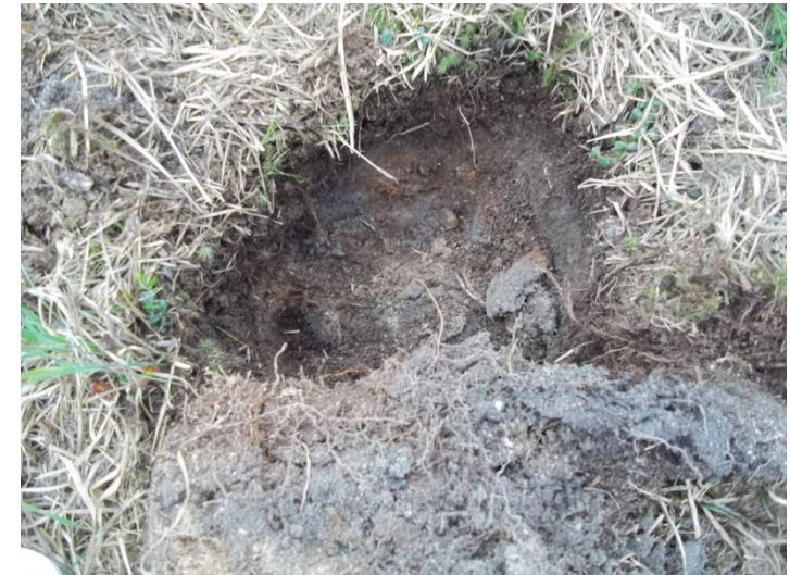
Test pit excavation for WABUSH3-SS26.
