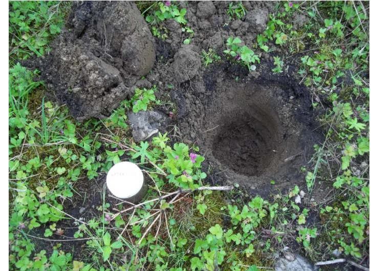
Test pit excavation for WABUSH3-SS1.
