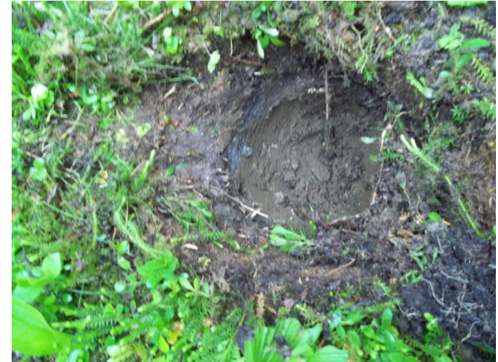
Test pit excavation for WABUSH3-SS20.
