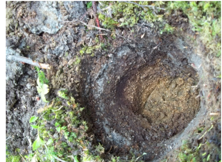
Test pit excavation WABUSH3-SS10.
