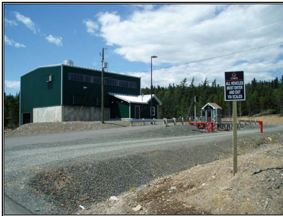
Figure 7-2: Pre-Engineered Building Housing a Tipping Floor, Trailer, Office, and Washroom
