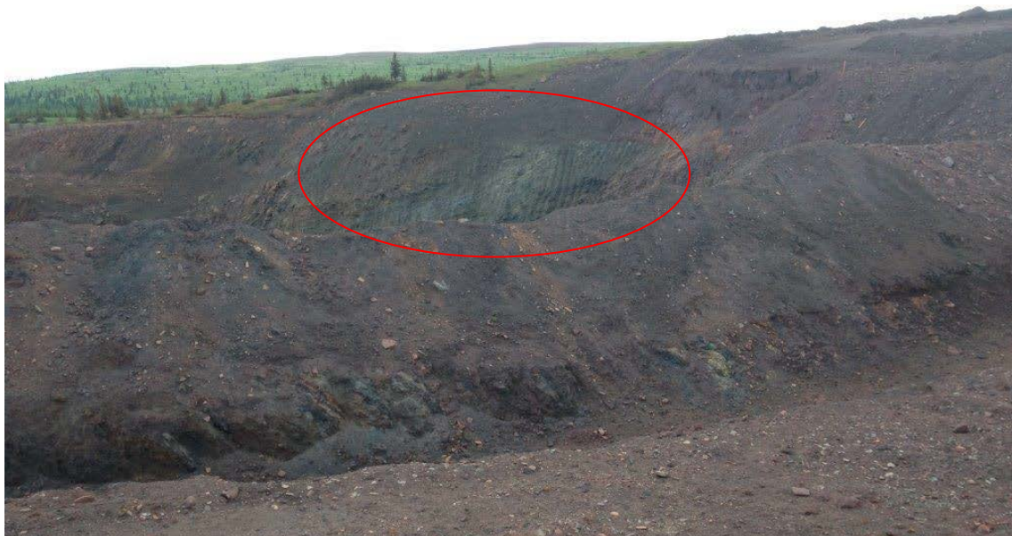
Figure 4-1: Photo showing excavator teeth marks in pockets of warm permafrost in Timmins 4N
