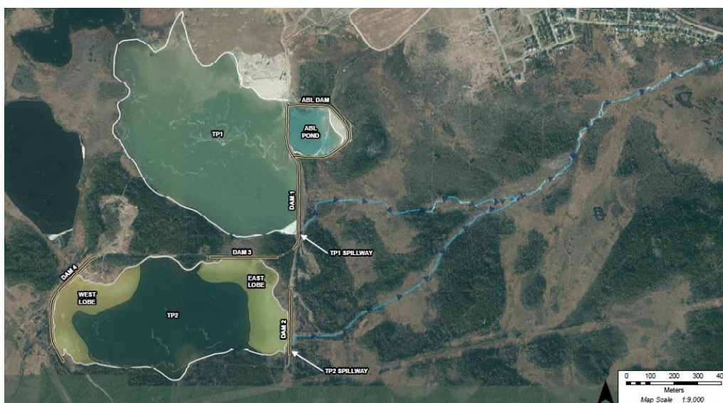
Photo i - Overhead View of Tailings Ponds and edge of Town (top right)
