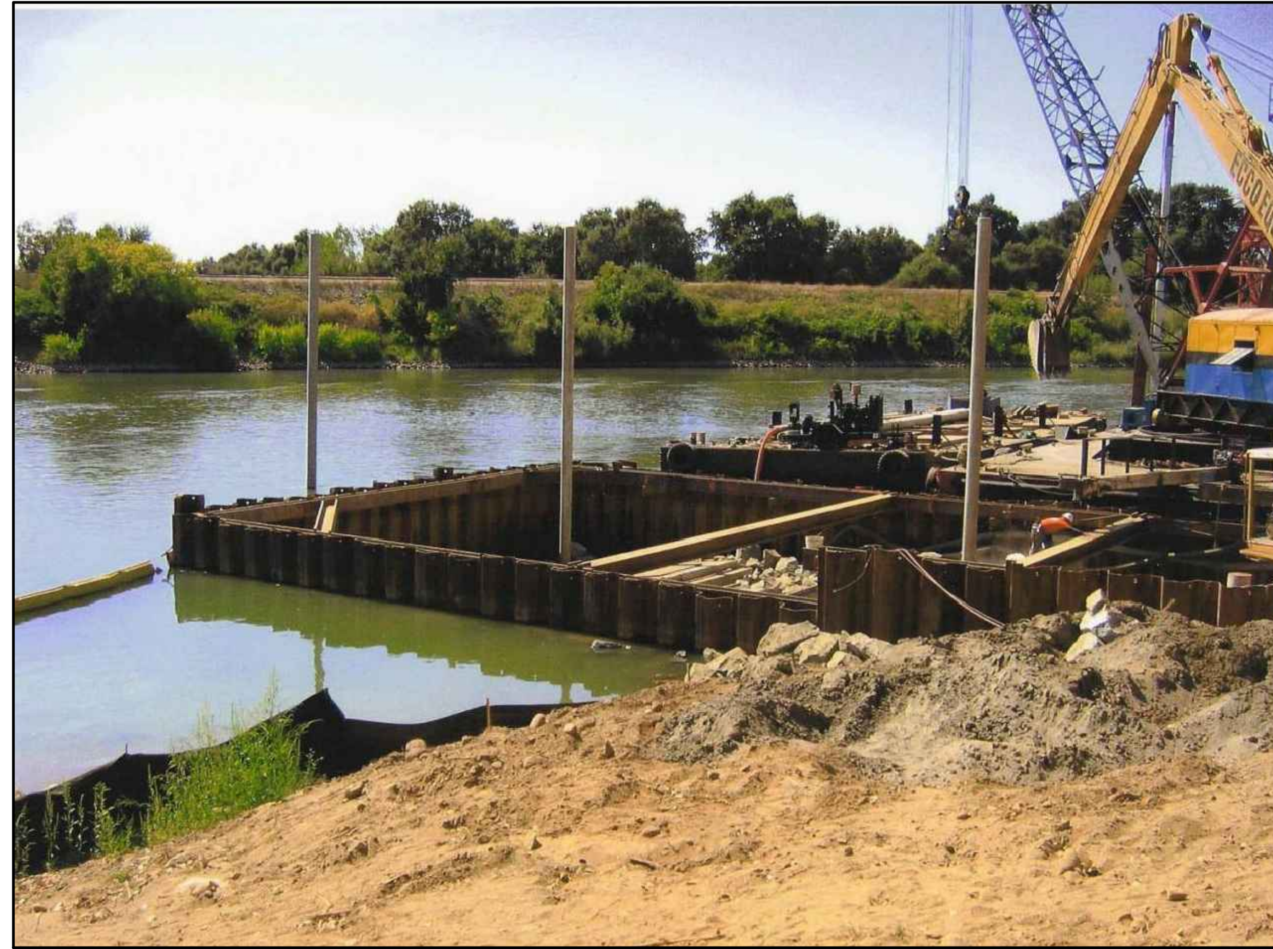
TYPICAL COFFERDAM SETUP
