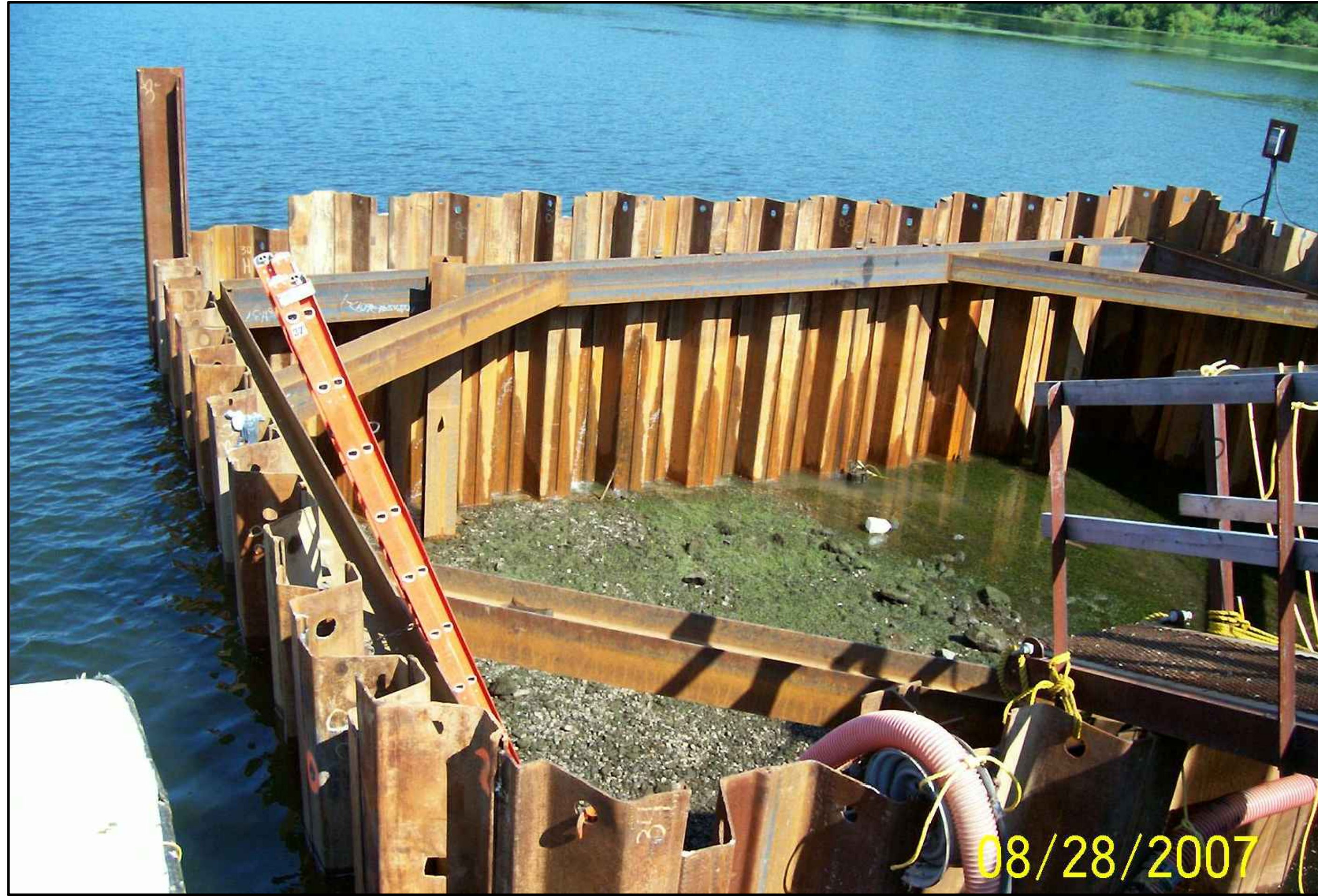
TYPICAL COFFERDAM SETUP
