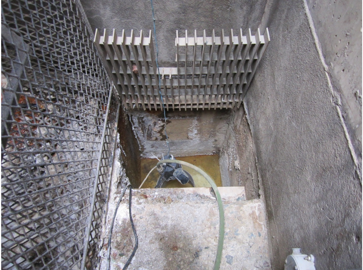
Photo 4 – Sump pump beneath ventilation hatch
