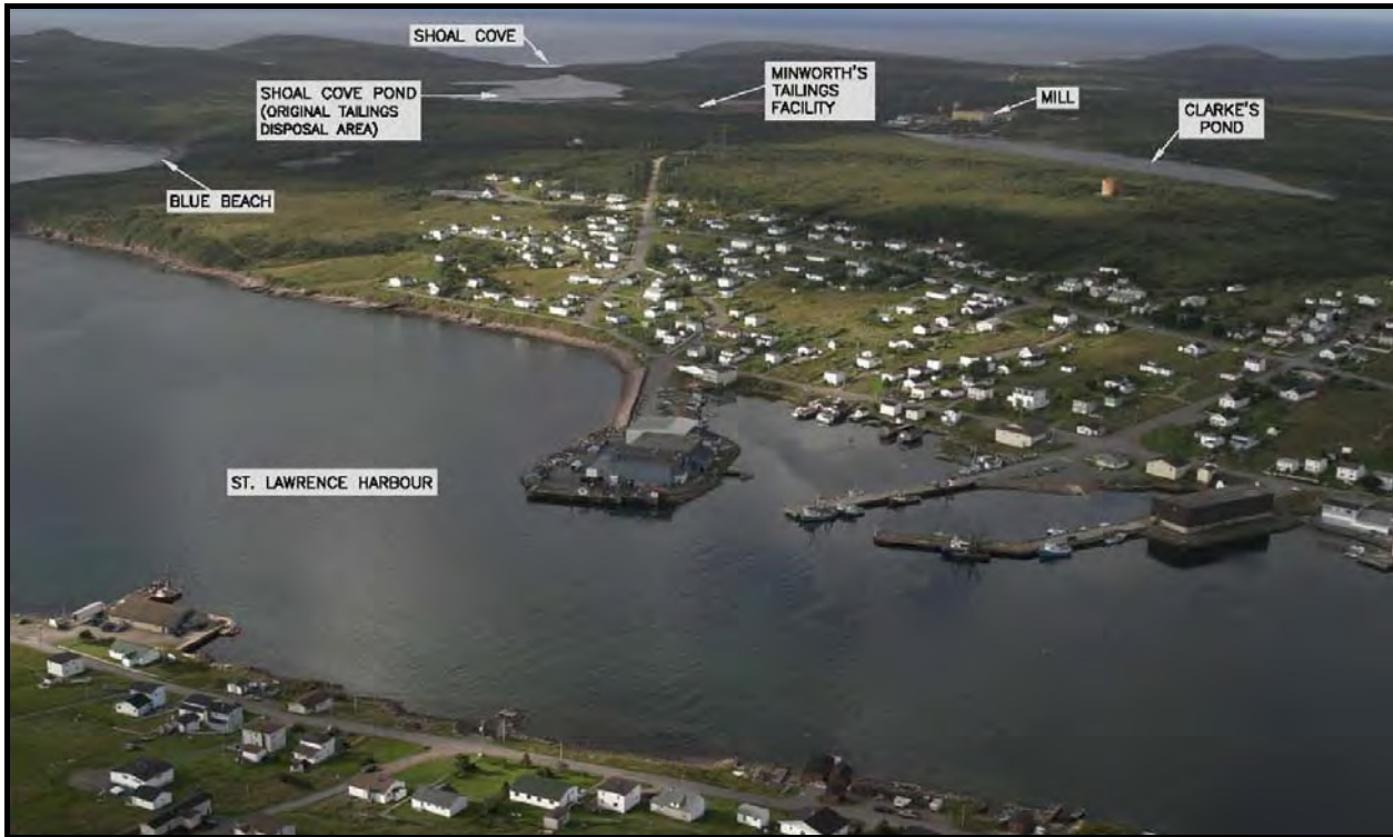
Figure 2-3: Aerial Image of Town of St. Lawrence and Project Site (original photo courtesy of DFO, BML 2009)
