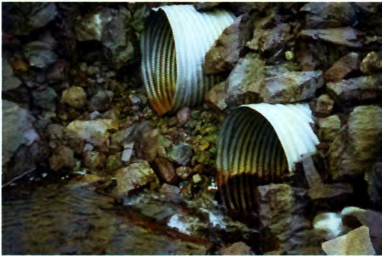
Figure 4.22 Multiple Culvert Installation
