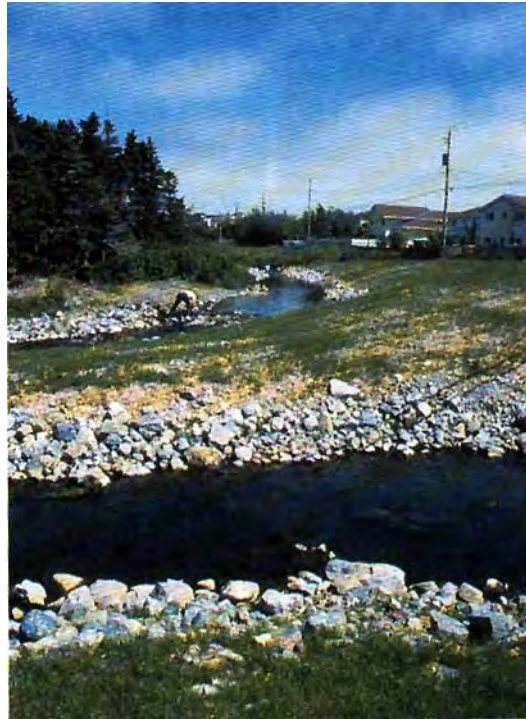
Figure 4.14 Rock riprap prevents erosion.
