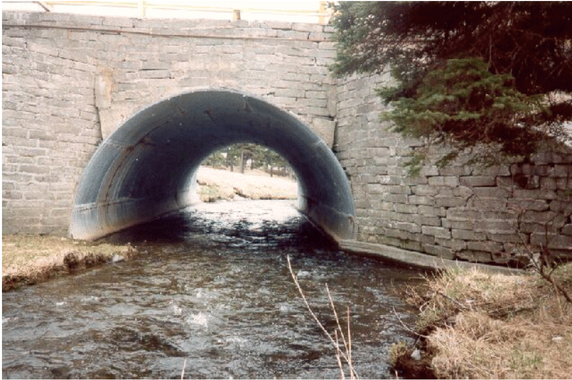
Figure 5.6 Pipe Arch Culvert with Masonry Headwall and Wingwalls
