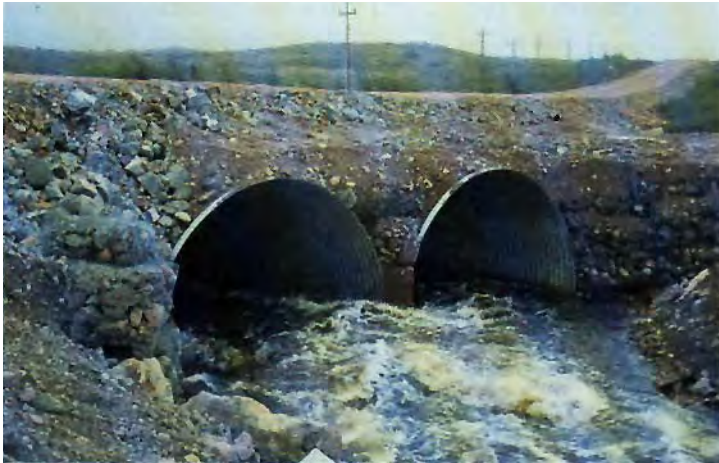
(a) Bottomless arch installation.
