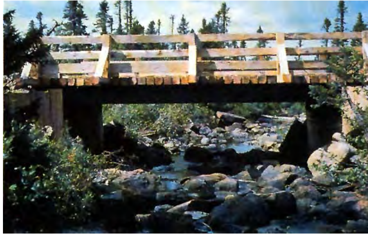
Figure 4.18 A well-designed bridge allows for a natural stream bottom at a crossing site.
