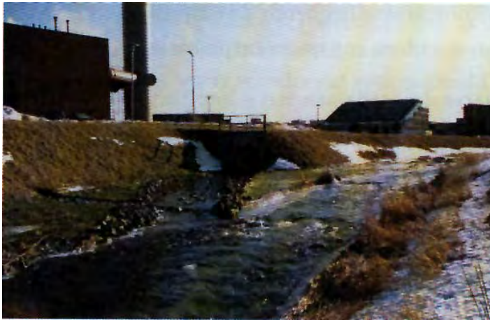
Figure 4.39 Storm drainage outlets should be connected to the receiving watercourse by a channel with orientation parallel to the flow of the receiving watercourse.
