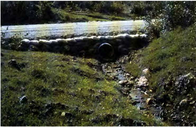
Figure 4.10 Cross drainage culverts and take-off ditches carry water away from the road and into surrounding vegetation.
