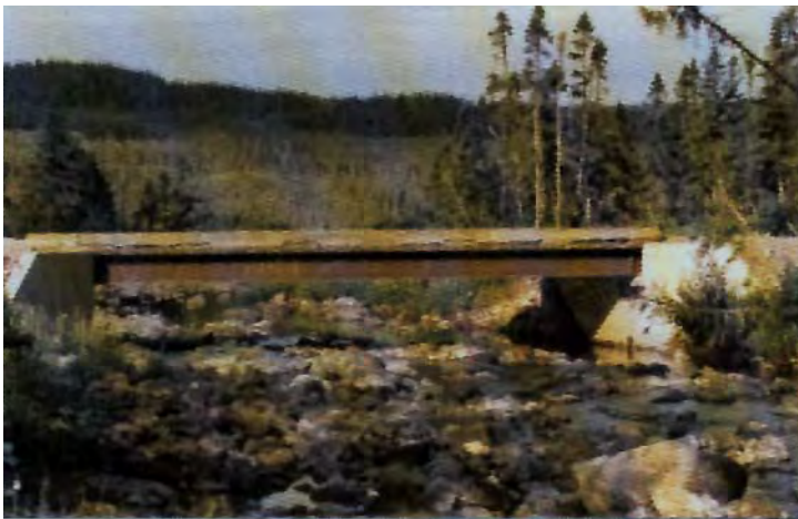
(b) Permanent bridge.
