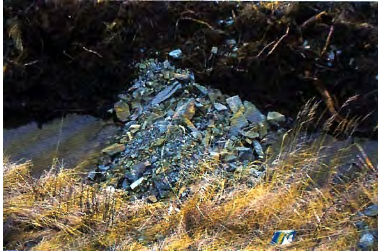
Figure 4.5 Check dams can be constructed from a variety of readily available materials, including rocks.
